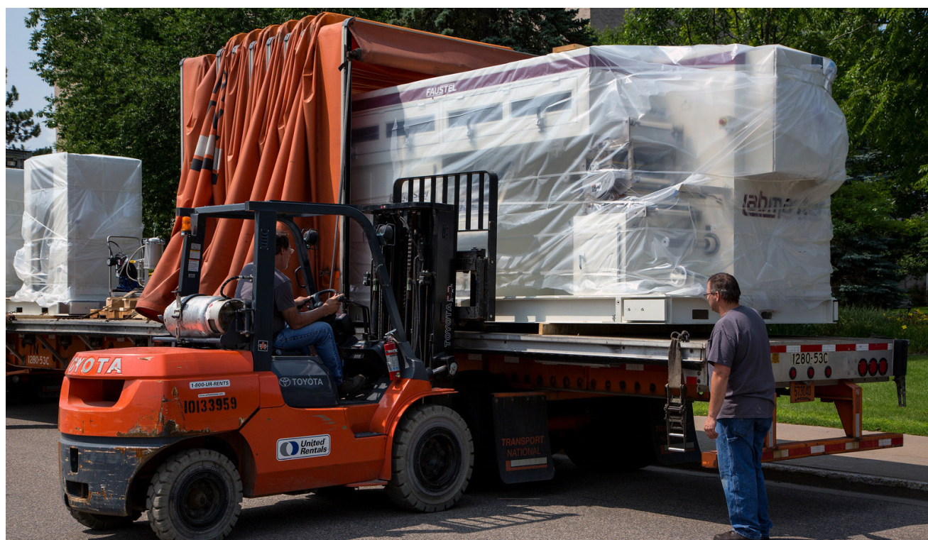
Steve Janisch and Tom Umbach of Faustel Corp. prepare to unload the main unit of the coating and laminating machine.
