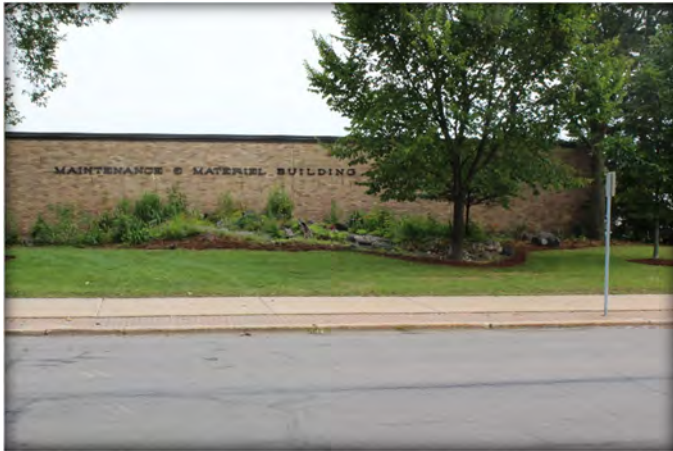
Maintenance & Materials Building
