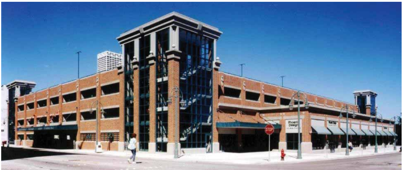
Stair tower articulated with use of materials. Ground level of ramp is lined with retail uses to bring to a pedestrian scale.
