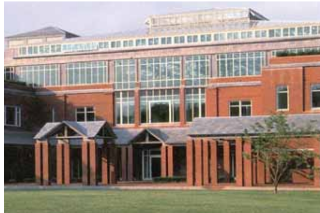
Material selection, combination, size, texture and color affect the overall building appearance.
