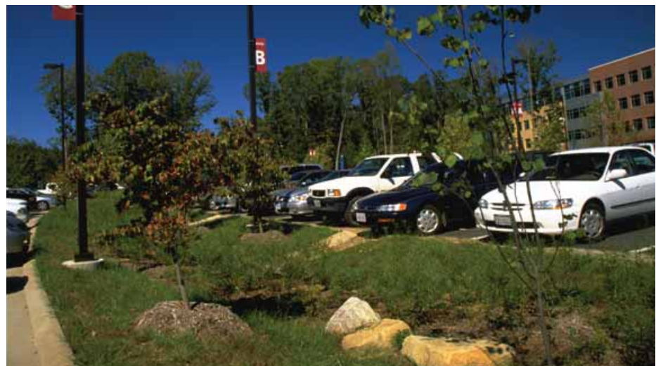
Bioswale allows for stormwater infiltration.
