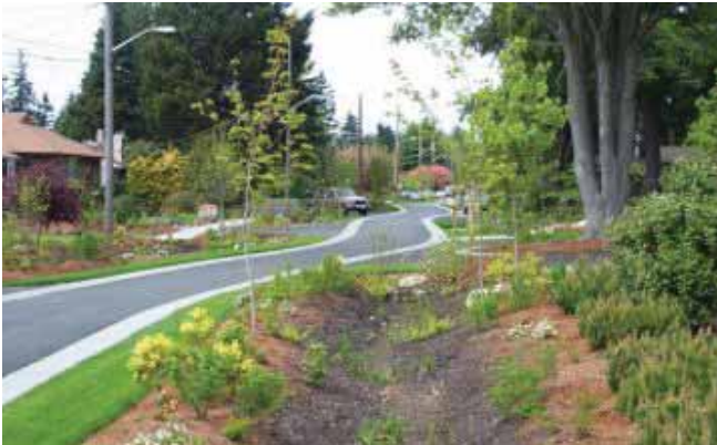
Planting islands with curb cuts allow for stormwater infiltration.
