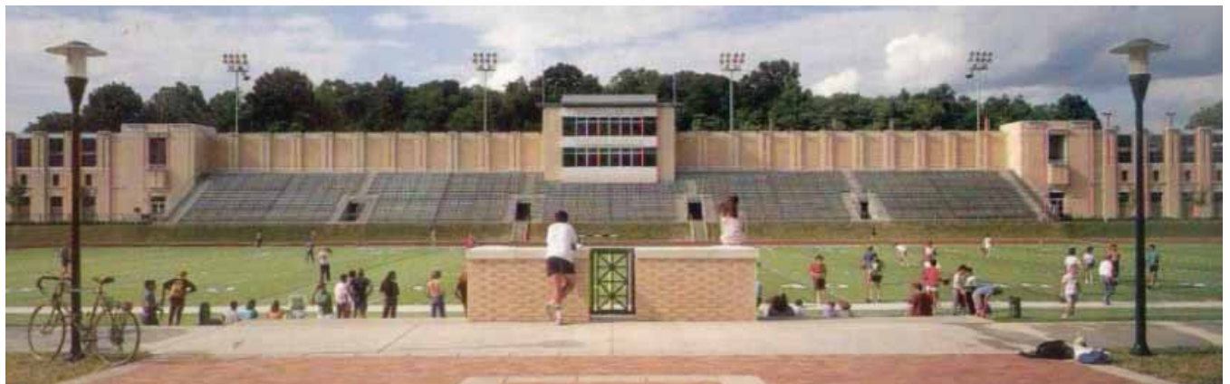
Sports complex uses material combinations and building articulation to reduce perceived scale of large buildings.
