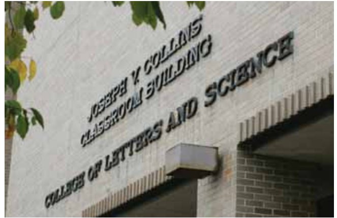
Existing building identification - building mounted
