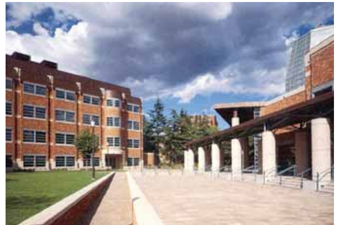
Articulated facade reduces perceived scale of large building.
