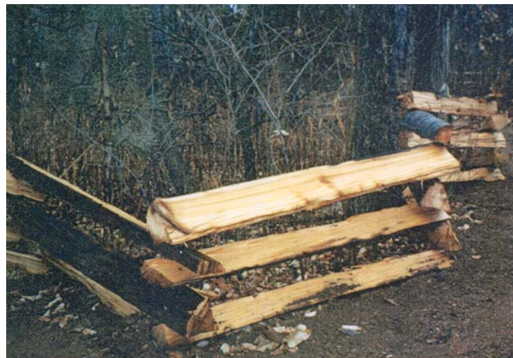
Oakfield Tech Ed students built this split rail fence made from old utility poles to embellish their nature trail.
