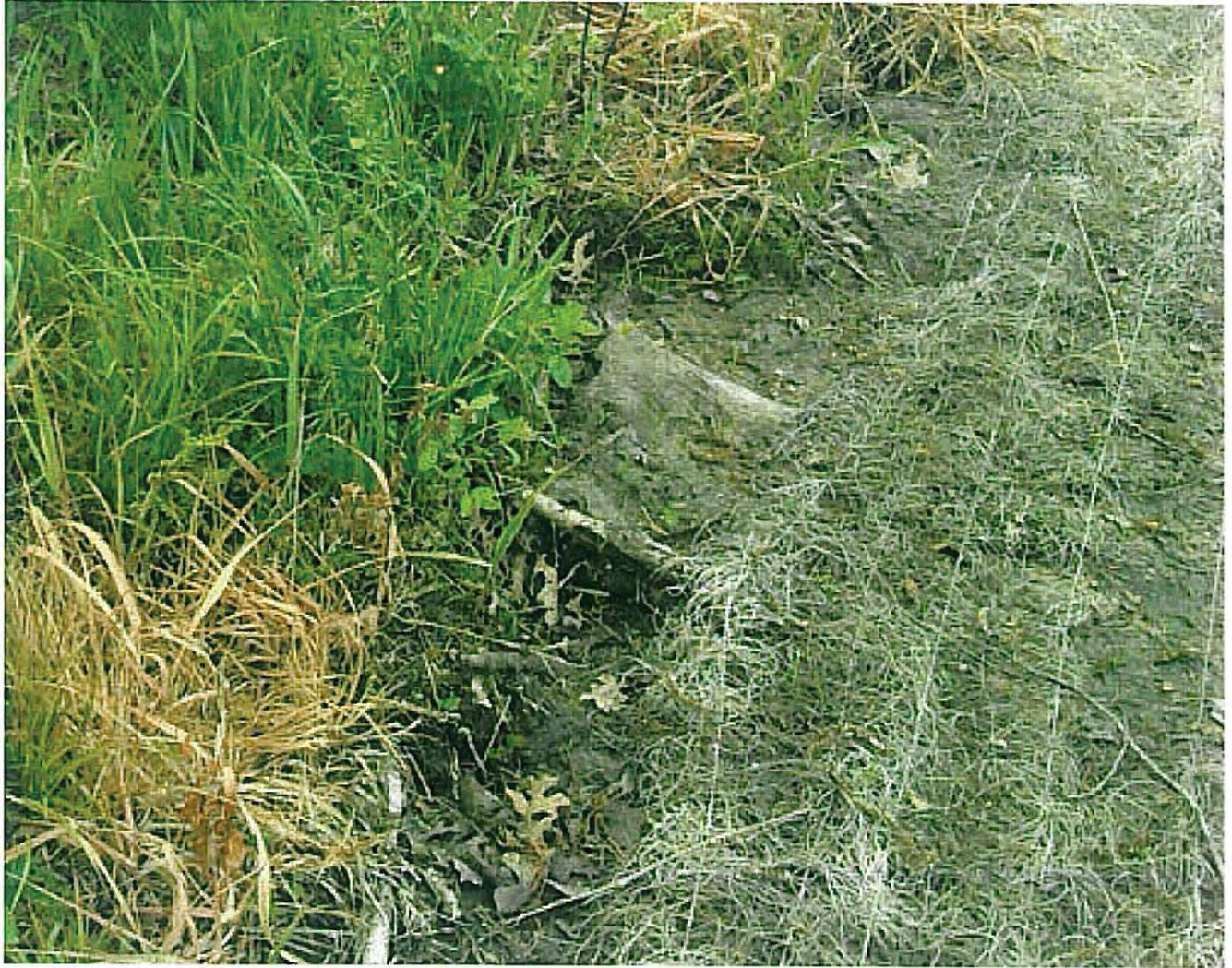
Photo showing the die-back of RCG from the previous application.
