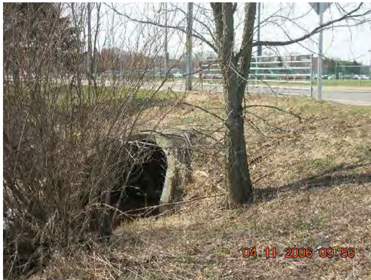
Figure 3-10 - Culvert where Moses Creek enters the underground system
