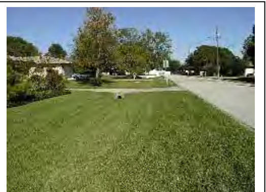
Figure 7-9 - Drainage Swale Source - www.altamonte.org
