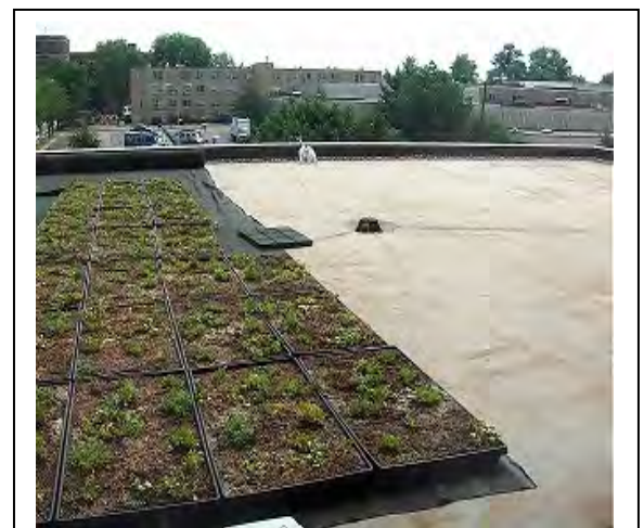
Figure 7-7 - Green Roof being constructed at UWSP Source: UW – Stevens Point
