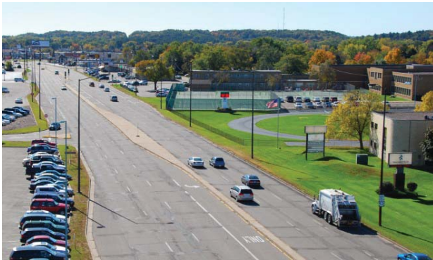
Figure P1 Highway 53 corridor in the City of La Crosse (top) reenvisioned as a green complete street (bottom).
