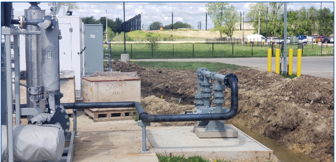
Photo 5: Pipeline injection of biogas from a Dane County Landfill, Dane County Public Works, Madison, WI
