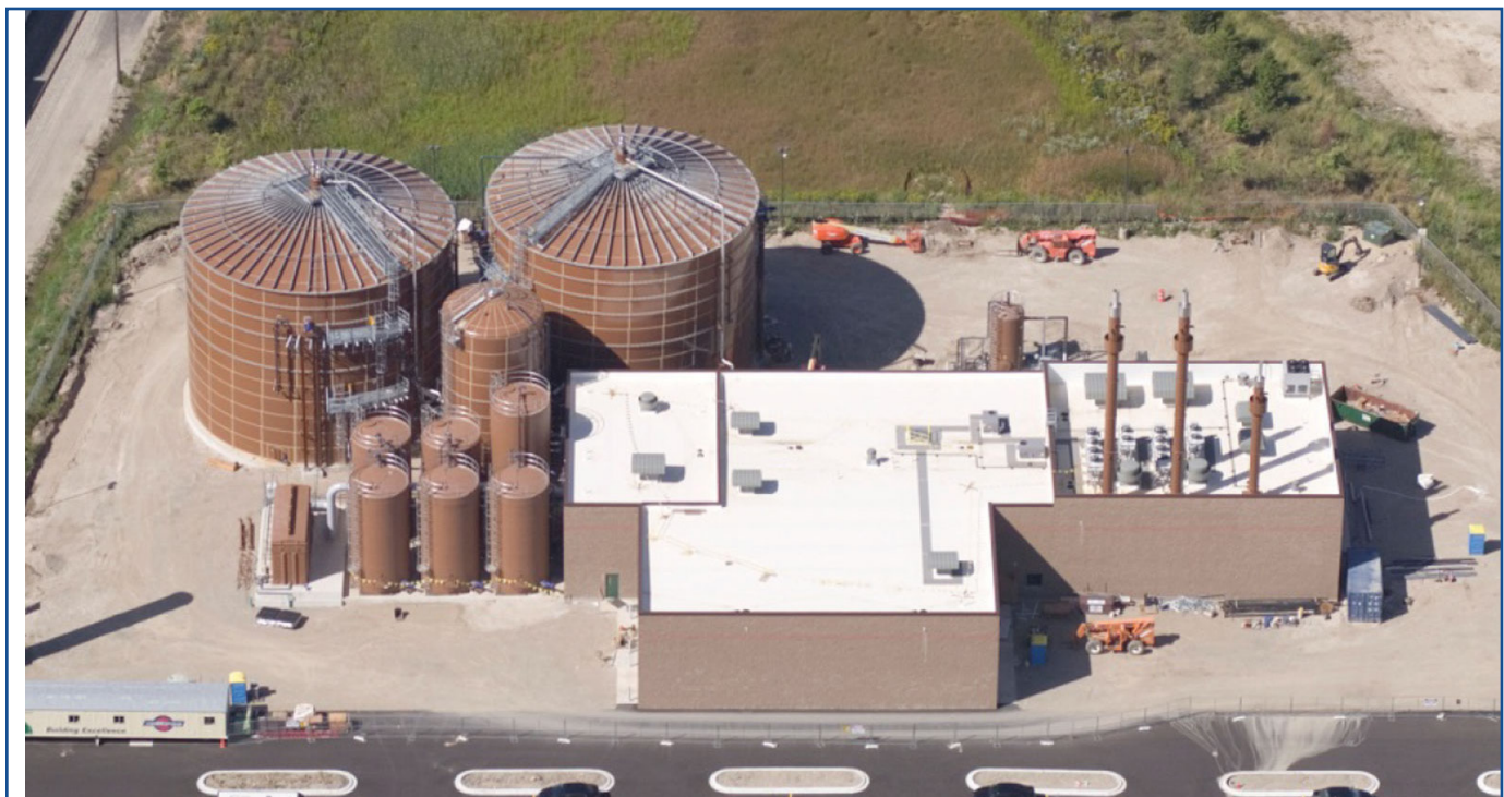
Photo 4: Food waste-to-energy biodigester facility, Forest County Potawatomi Community Renewable Generation, LLC,
