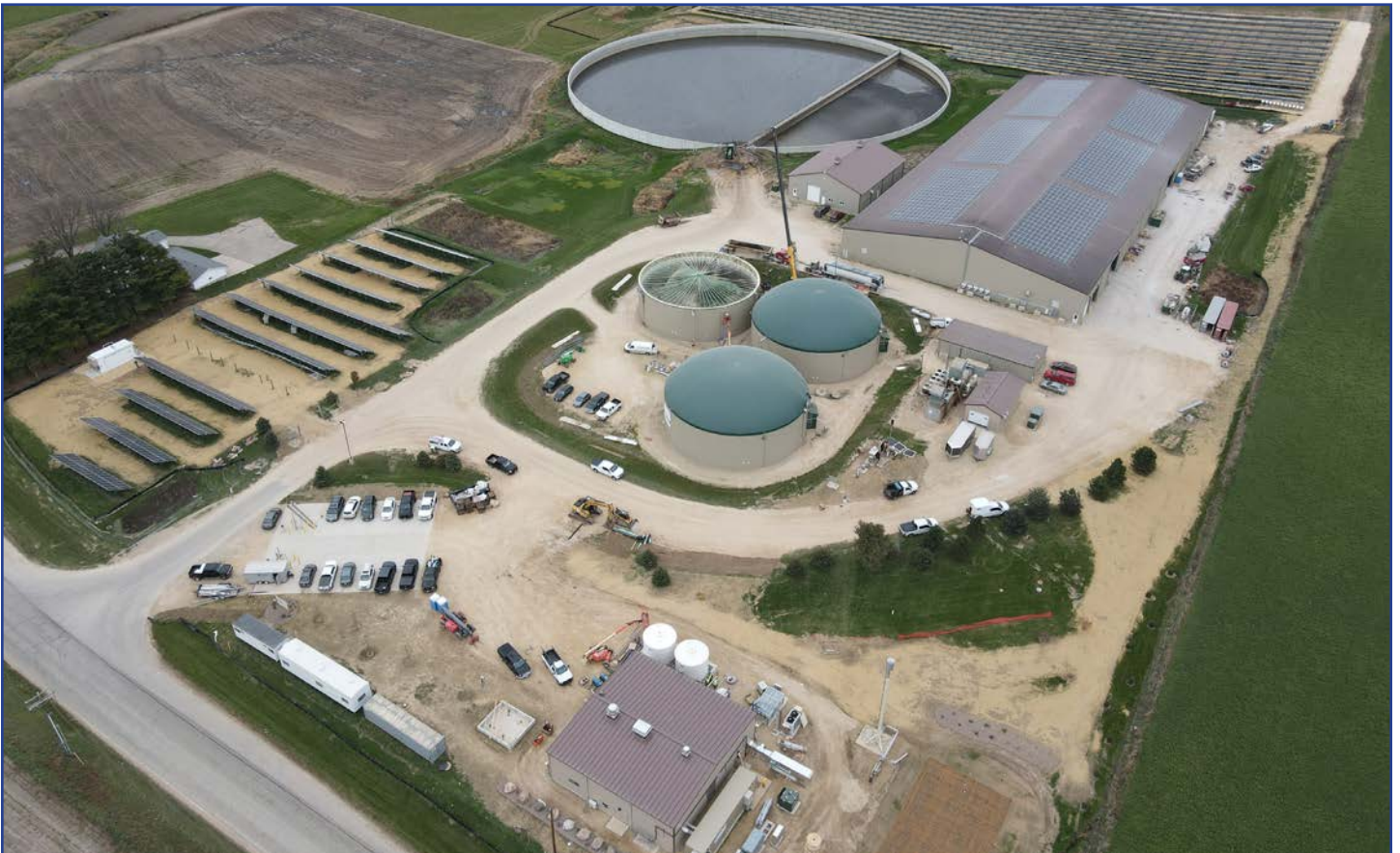
EnTech Solutions Middleton digester facility, Town of Springfield, Wisconsin
