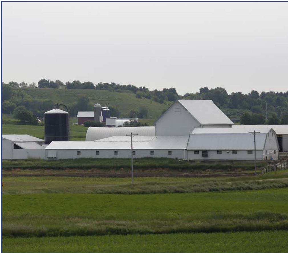
Zeigler Dairy Farms across from EnTech Solutions transports manure via pipeline to the digester
