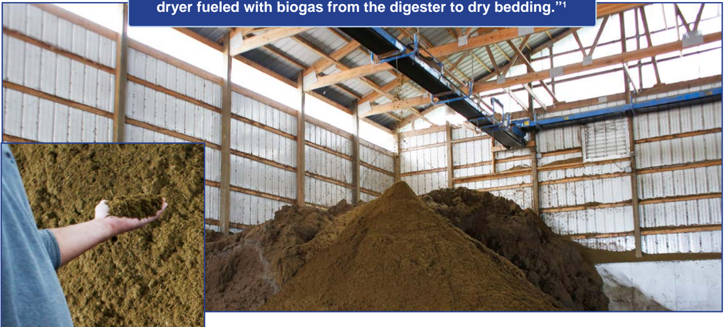
Left: Digestate screw press; Right: Digestate dryer; Bottom: Dried digestate delivered via conveyor belt from the dryer
