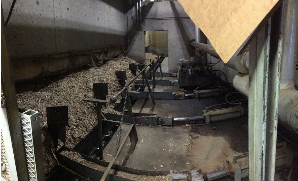
Photo 1: Wood Chip Auger Delivery System For Barron School District's Wood Boiler Heating System, Barron, WI.
