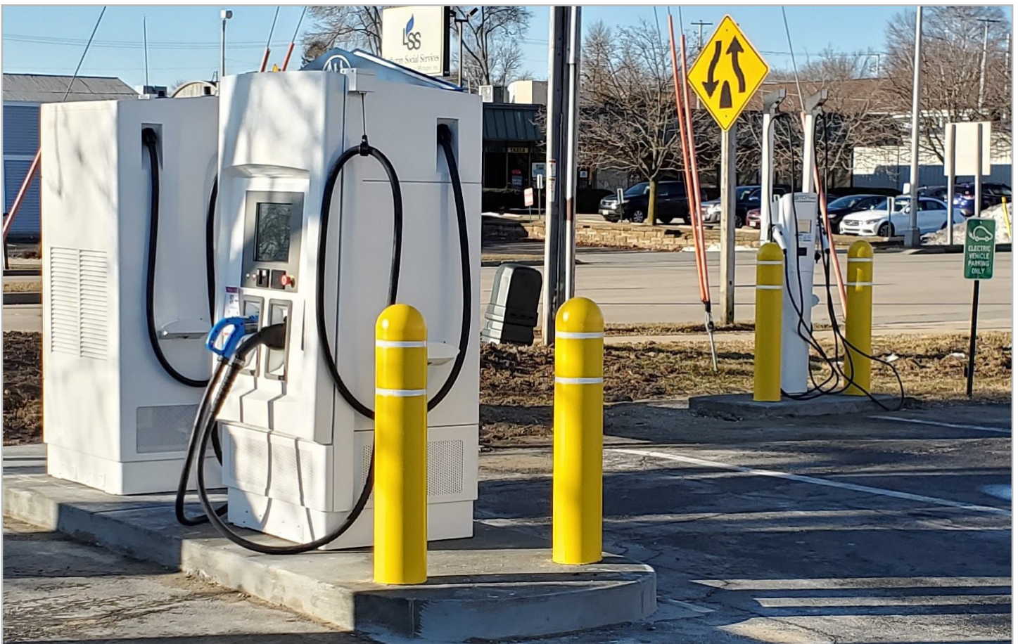
Photo 7: Level Two and DC Fast Charging Station, Park Village Shopping Center, Beaver Dam, Wisconsin
