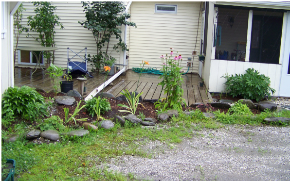
Roof Top Disconnection and Rain Garden
