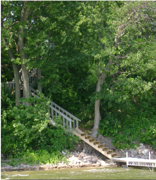
Vegetation surrounding a stairway: Mature vegetation above and around this zig-zag stairway protects the slope from erosion.
