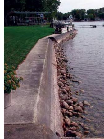
Figure 2. Bulkhead seawalls reflect wave energy and create barriers for many aquatic animals.
