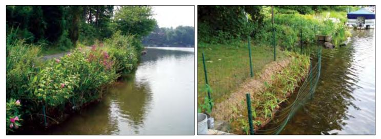
Figure 2. A re-established vegetated shoreline (1) and a newly installed and planted coir log (r).
