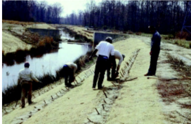
Figure 16-9b Installing live stakes in live fascine system (Robbin B. Sotir & Associates photo)
