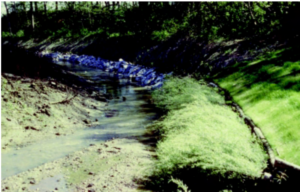
Figure 16-15c An established live cribwall system
