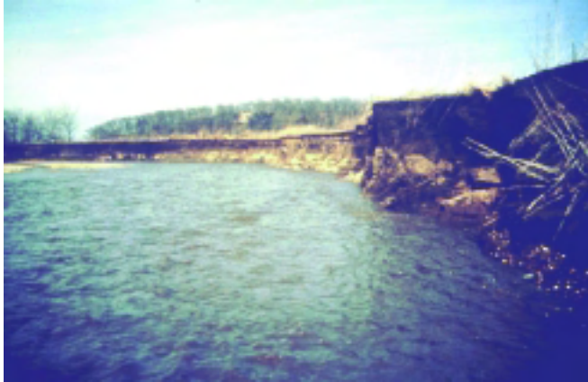
Figure 16-25a Pre-construction streambank conditions (Don Roseboom photo)
