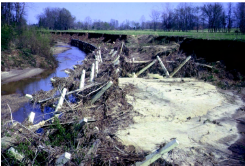
Figure 16-31 Concrete jack system several years after installation
