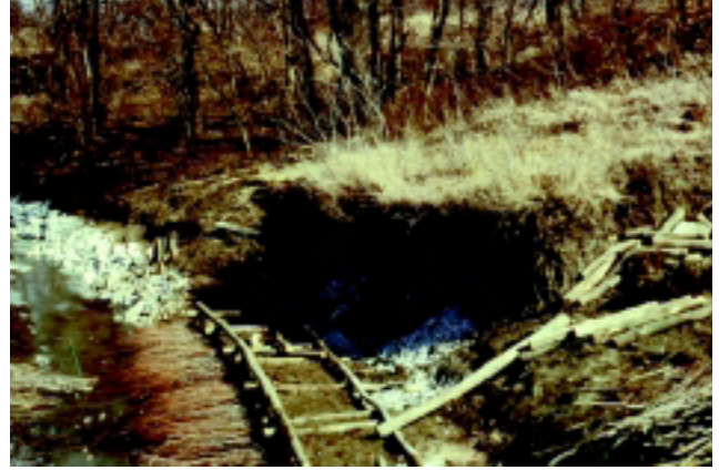
Figure 16-15b A live cribwall during installation
