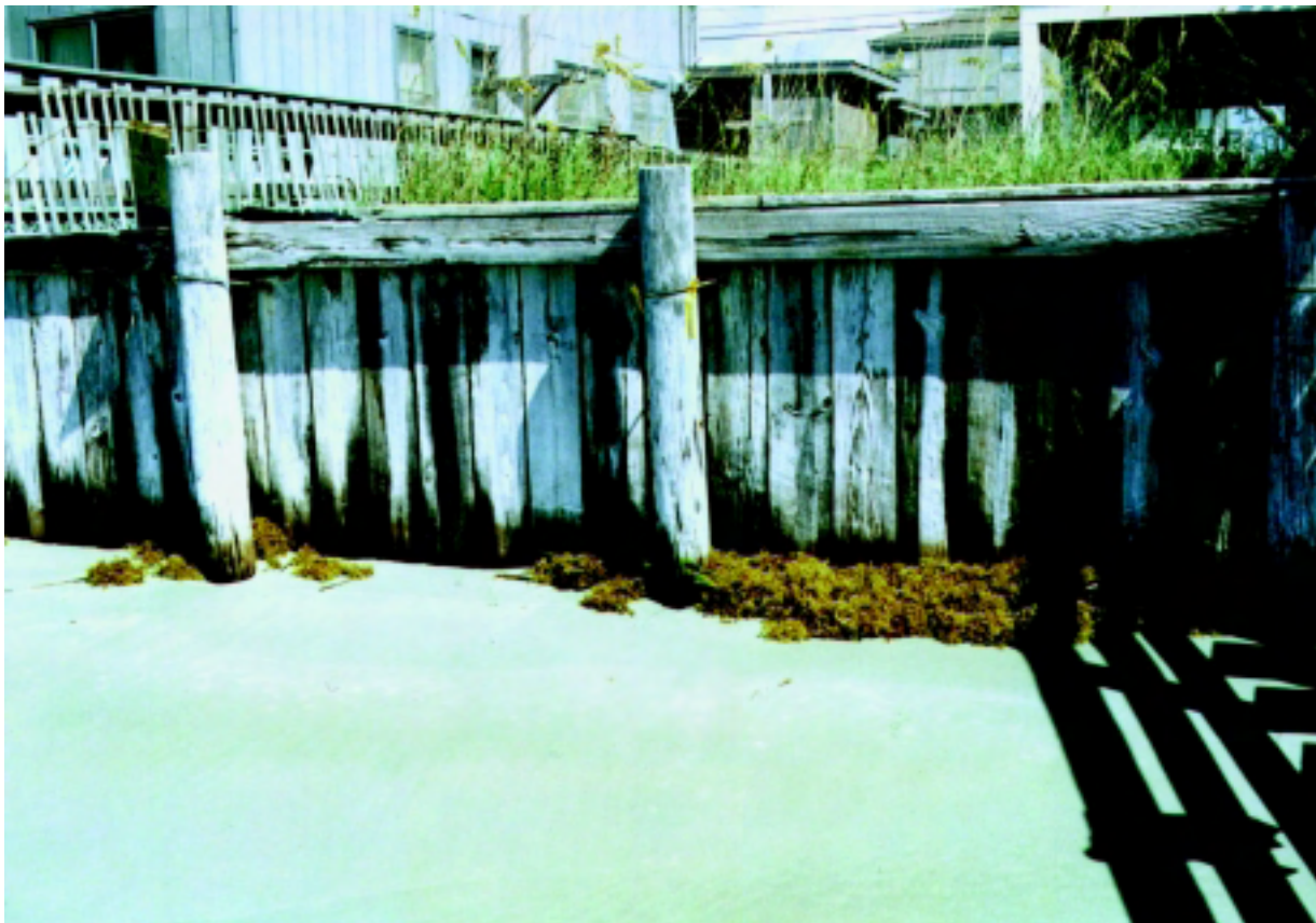
Figure 16-46 Timber bulkhead system
