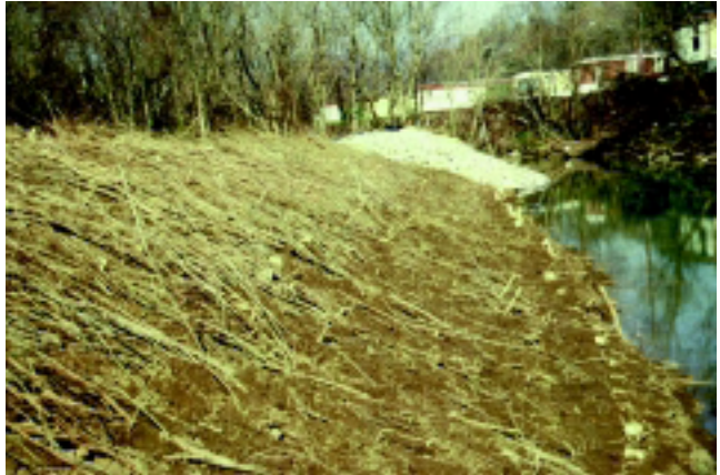
Figure 16-19b An installed brushmattress system (Robbin B. Sotir & Associates photo)
