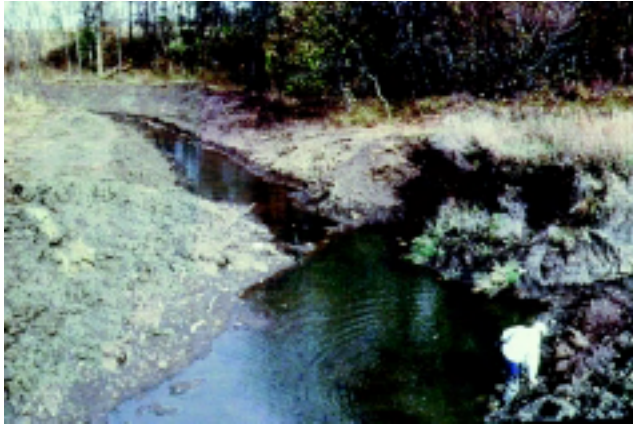
Figure 16-15a Pre-construction streambank conditions
