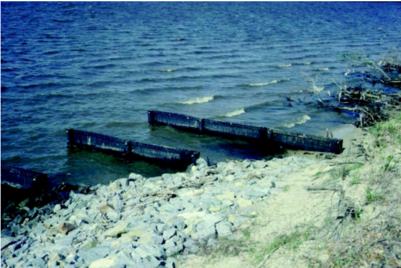
Figure 16-45 Timber groin system
