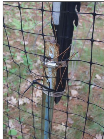
Clamps can be used to attach extender poles
