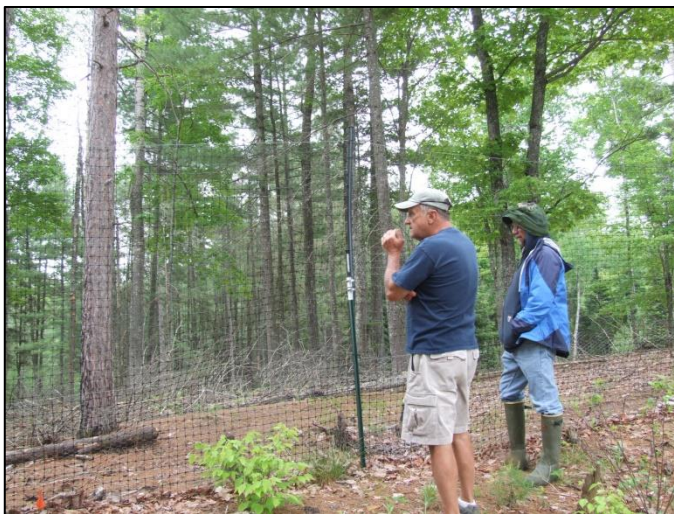
T-post example with extender pole and shock cord at the top
