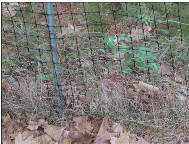
Line of chicken wire at base of fence
