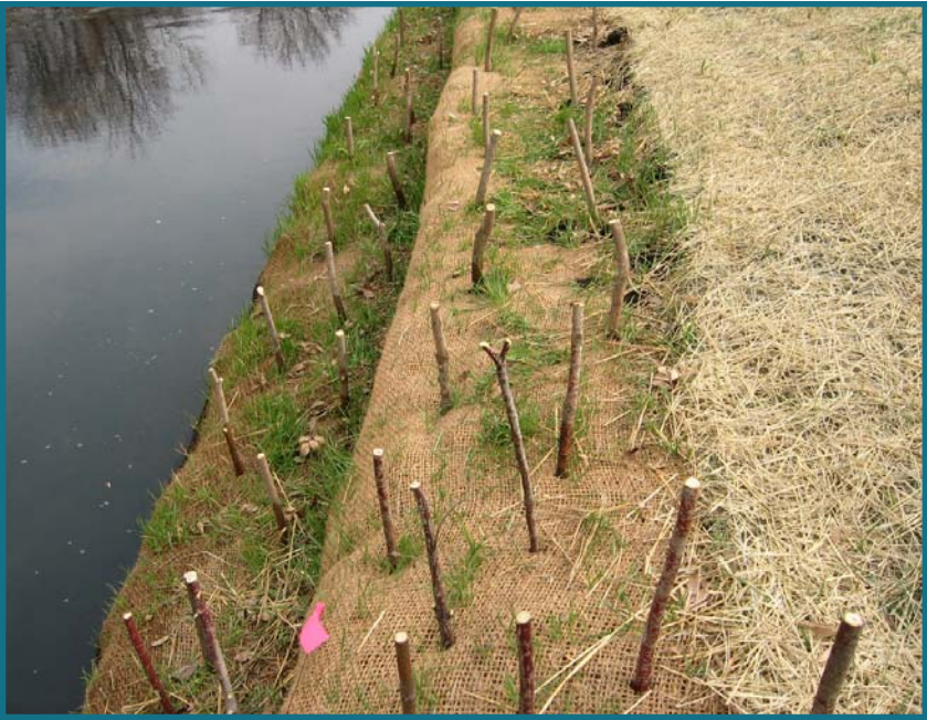
Figure 4-9. Live stake plantings along the Vermillion River, a state recognized trout stream, in rural Dakota County.
