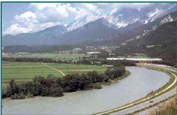
Figure 1-4. A soil bioengineered riparian bank using deep live posts in the Alps of Europe that is over 100 years old. Schiechtl and Stern 1994
