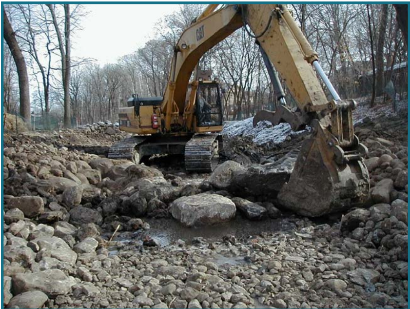
Figure 2-15. Rock vane installation. Pike Creek, Maple Grove, MN
