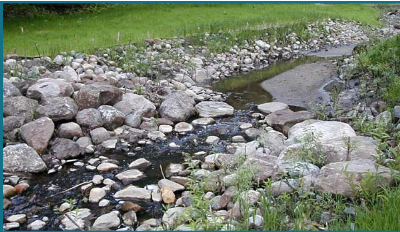
Figure 2-16. Rock vane and riffles after soil bioengineering construction.
