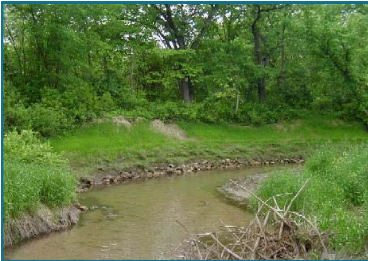
Figure 4-4. Before and after soil bioengineering stabilization with a vegetated reinforced soil stabilization (VRSS) system.
