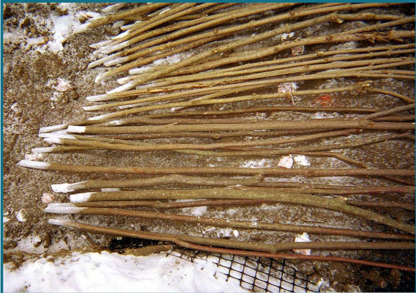
Figure 2-5. The basal ends of brush bundle live cuttings are dipped in rooting hormone before installation.
