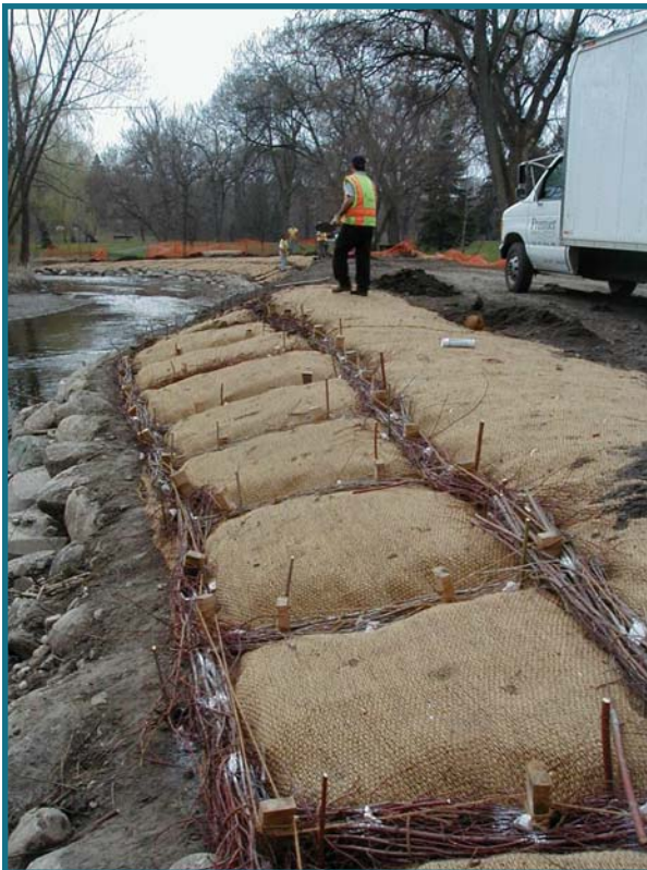
Figure 2-23. Vegetative geotextile including fascines and live stakes. Minnehaha Creek, Minneapolis
