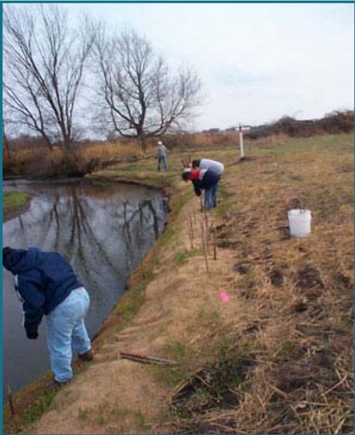
Figure 4-8. Planting soil bioengineering live stakes, in the dormant season, at the Vermillion River .
