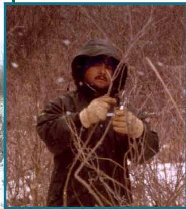
Figure 2-30. Harvest and transport of dormant willow stakes.
