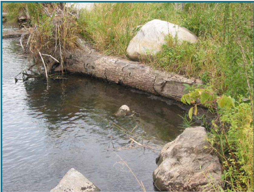
Figure 2-18. Rootwad installed in stream. Washington County, MN.
