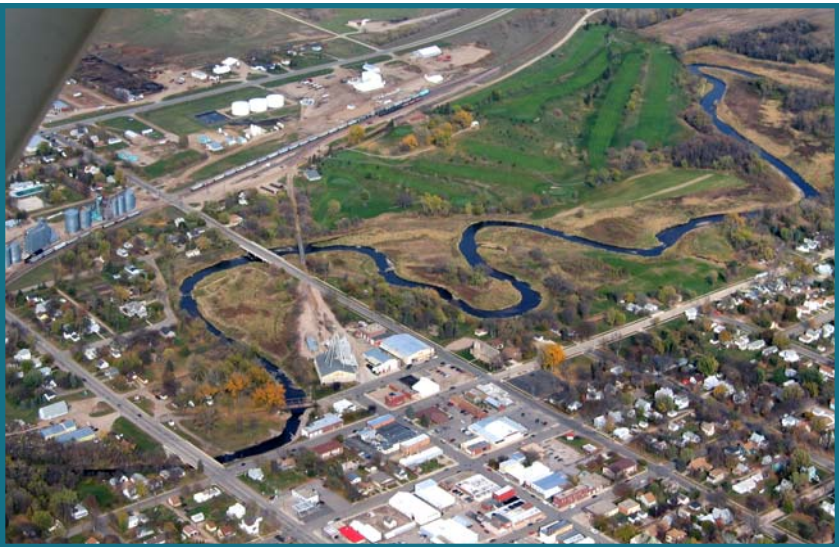
Figure 4-1. Dam removal and natural channel construction restored ecological and hydrological function to this stretch of the Pomme de Terre River in Appleton, MN. Photo courtesy of Luther Aadland, MN DNR.
