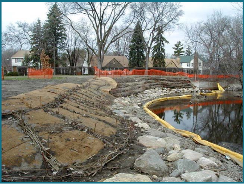
Figure 4-6. Minnehaha Creek during soil bioengineering construction.
