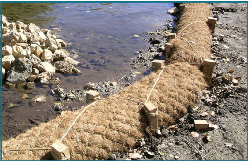
Figure 2-11. Fiber rolls after installation on a lake shore.
