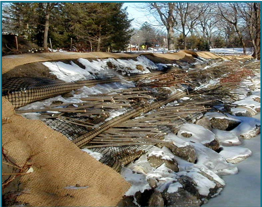
Figure 2-25. Vegetated reinforced soil stabilization planting. Minnehaha Creek, Minneapolis
