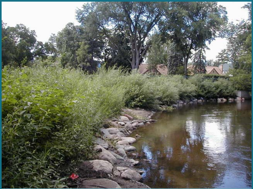
Figure 4-7. Minnehaha Creek two years after soil bioengineering installation.
