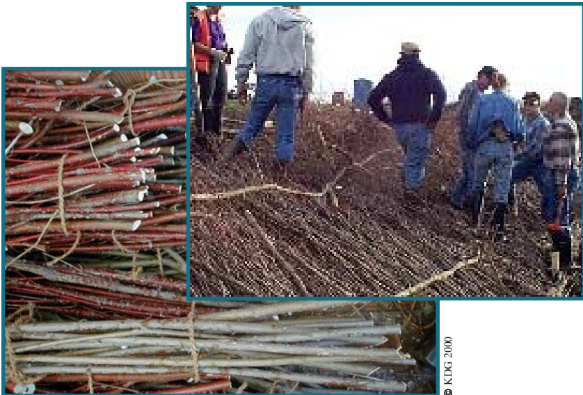
Figure 2-7. Live branch cuttings (LEFT) and brush mattress installation (RIGHT).
