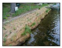
Photo 14. Planted double-level biologs and backfilled slope – Grass Lake.
