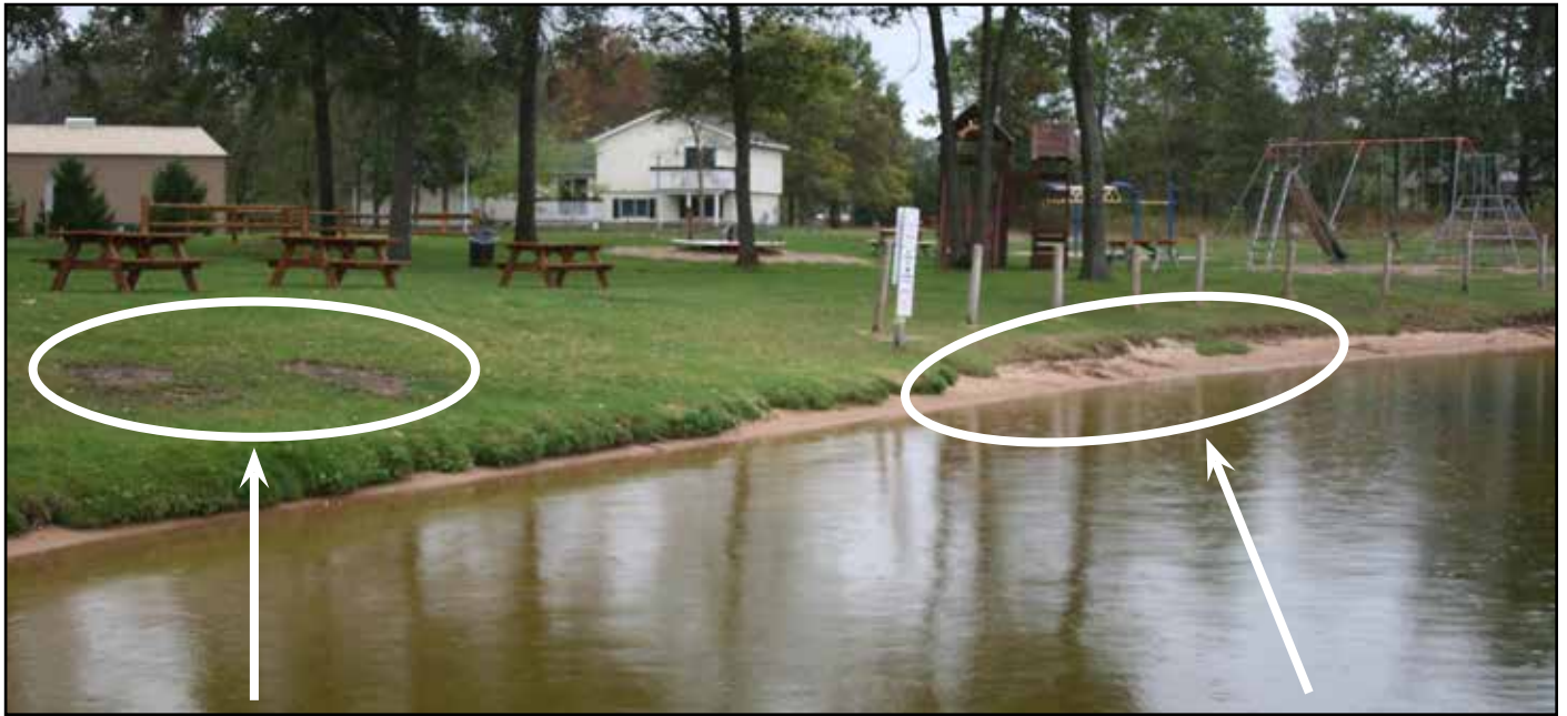
Evidence of overland runoff erosion coupled with heavy foot traffic.
