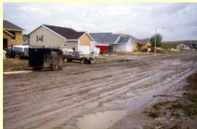
Urban construction sites
