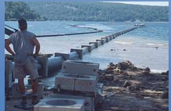
Pump out water
