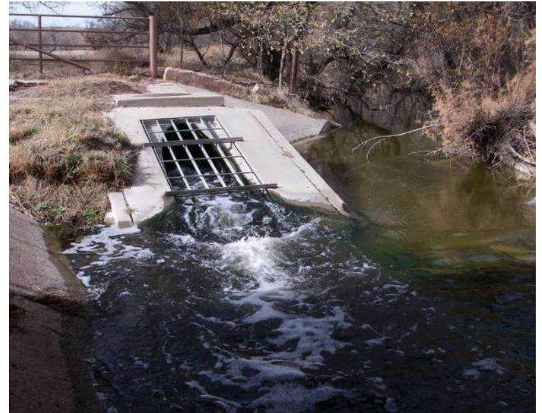
Municipal & Industrial Waste
