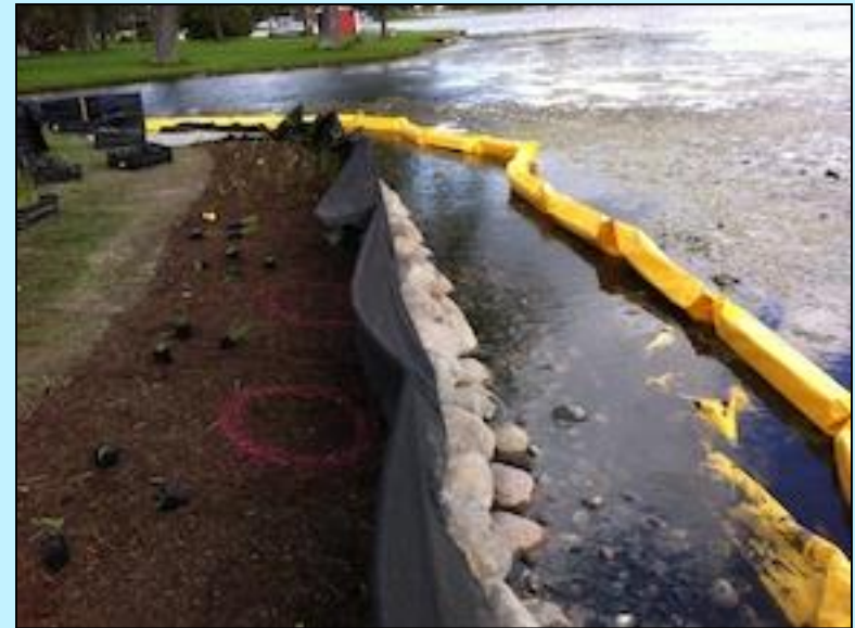
Beginning Landscaping – erosion barriers
