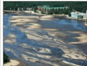
Lake Delton in Sauk County empty after CTH A failure. (June 2008)
