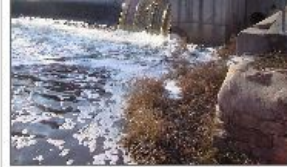
The Clarks Mill Dam, Town of Cato, Wisconsin
