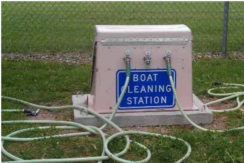
Green Bay – low pressure wash
