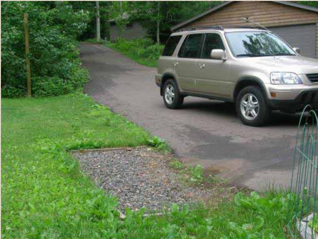
Rock Infiltration Pit
