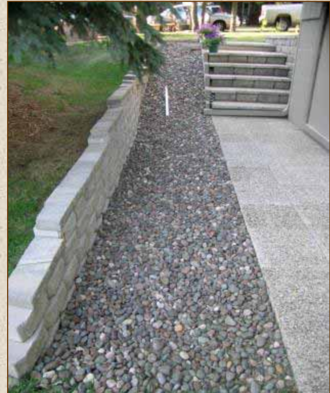
Rock Infiltration Trench
