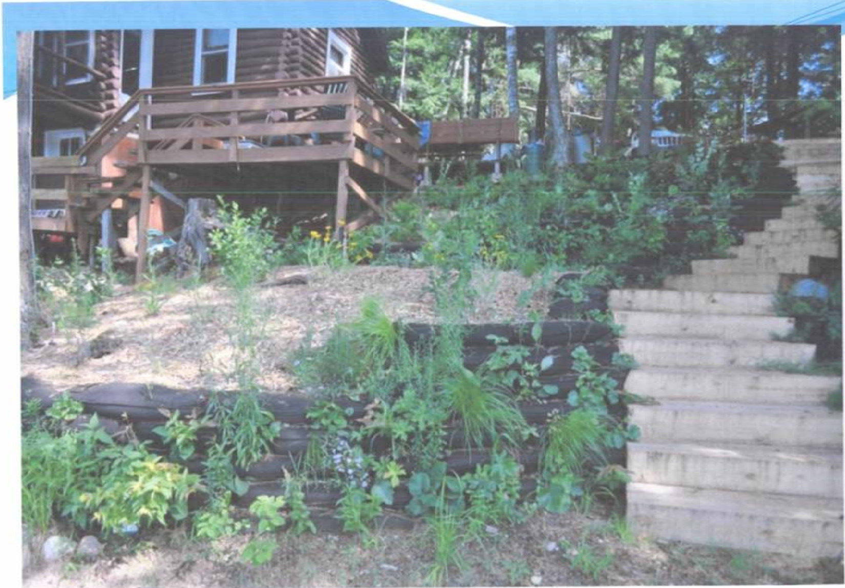
Vegetated Retaining Walls - Geotextile Bags (After)
