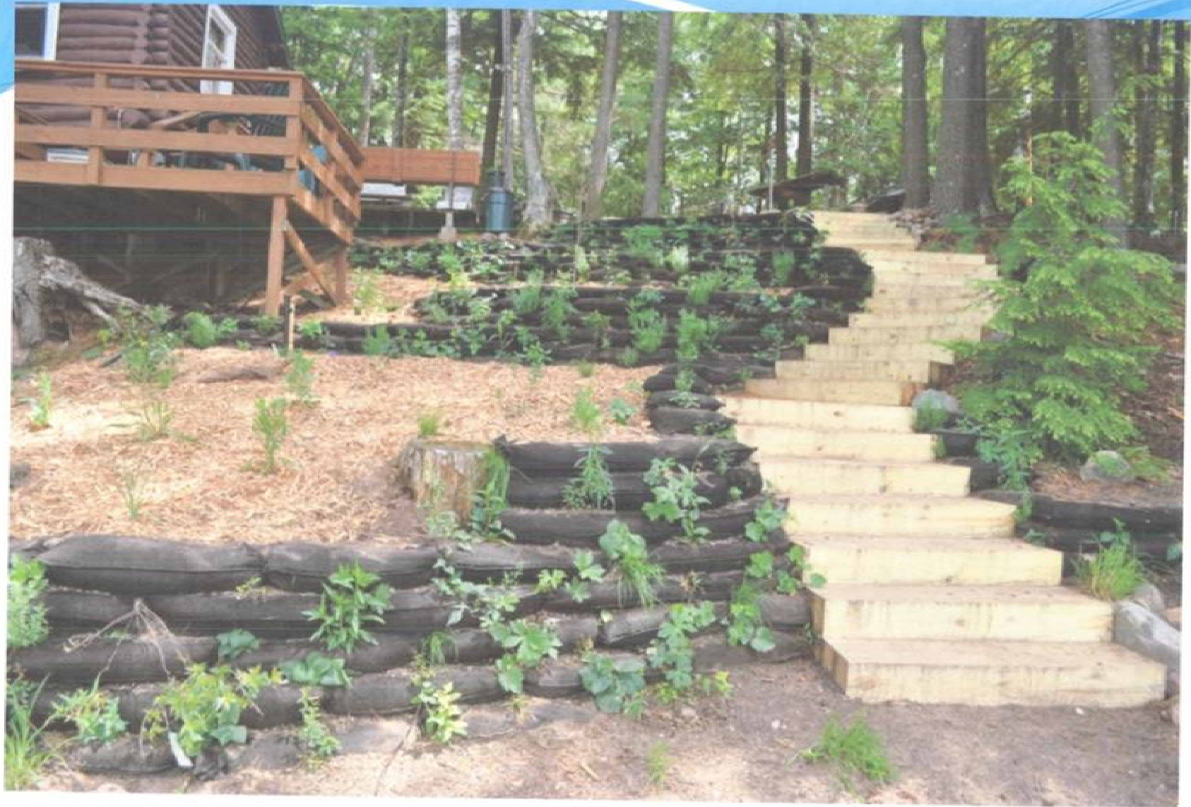
Vegetated Retaining Walls - Geotextile Bags (Install)
