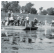
Applying chemical treatments to Lake Monona
