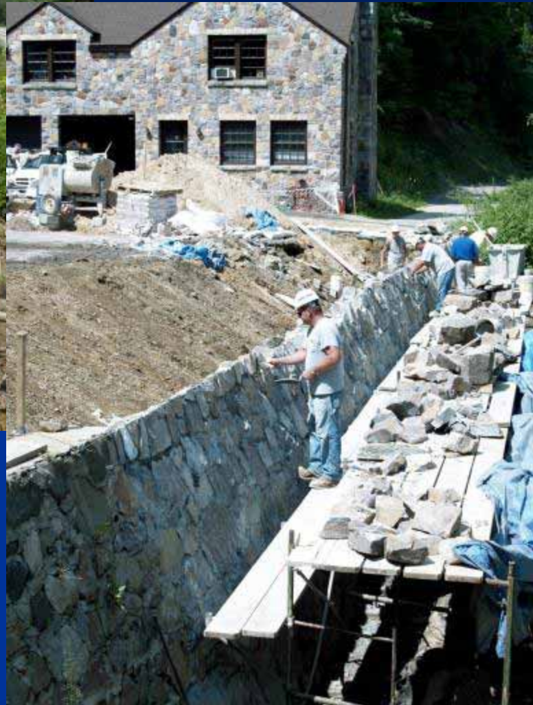
"replacement-in-kind" wall repairs in progress
