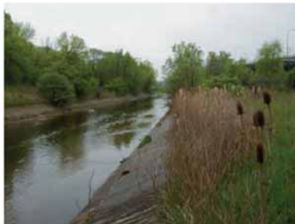
PRE-CONSTRUCTION SHOWING CONCRETE LINED STREAMBED AND STREAMBANKS
