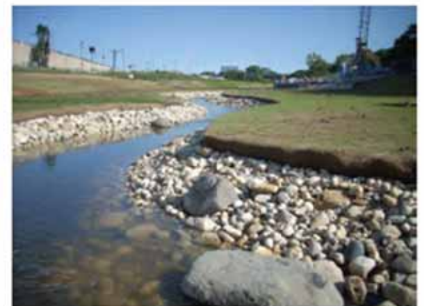
POST-CONSTRUCTION SHOWING RESTORED FLOODPLAIN CONNECTIVITY AND STREAM CHANNEL: 2009
