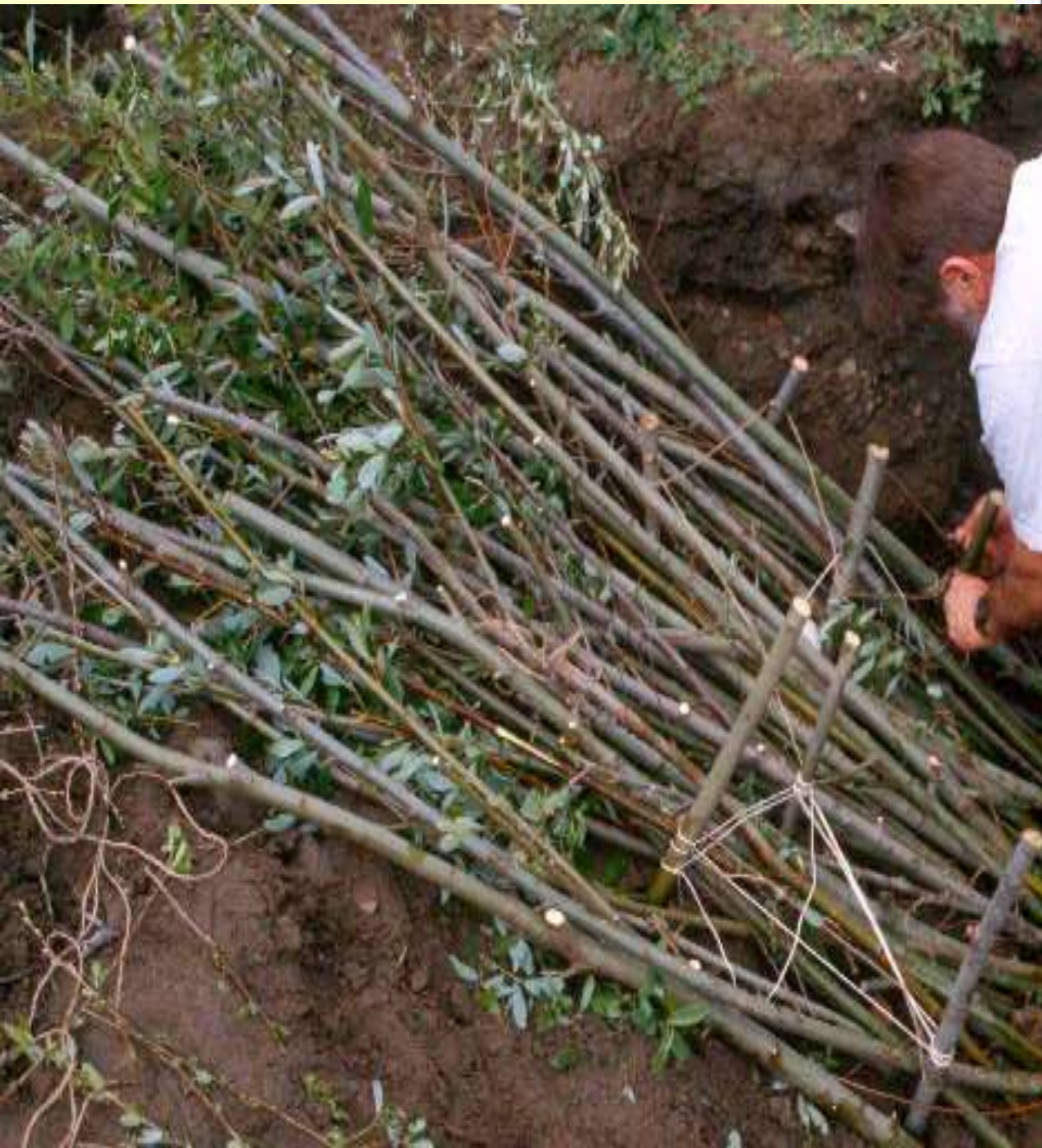
Step 1: Excavate trench and grade bank.
