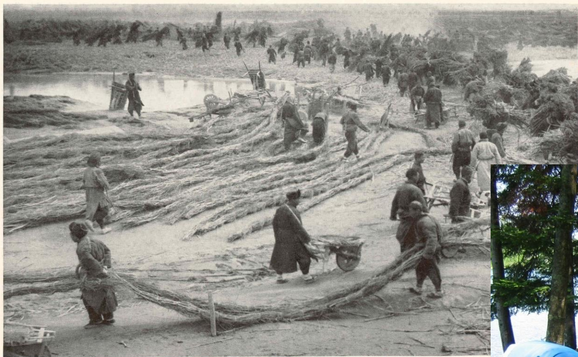
Swarming Along the River Bank Like Ants, Coolies Drag Long Strands of Woven Willow Sticks to the water's edge. Others carry packs of kaoliang stalks to the water's edge. Both materials rot in the water after a few years. Then new stacks are placed on the riverbank and the decayed mass is pushed into the mud on the river bottom. Often the entire construction is destroyed when the current scours out the mud.
