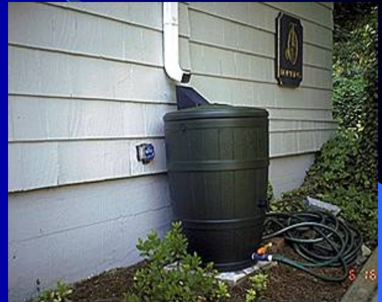
A rain barrel is used to collect rooftop runoff using a gutter/downspout system
