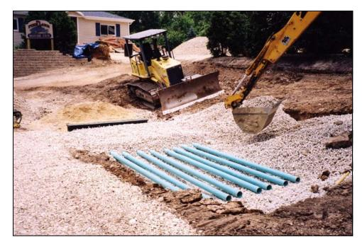
Example of a co-operator at a commercial site utilizing a subsurface retention system to collect and treat stormwater runoff thereby improving the quality and reducing the quantity of runoff entering Pike Lake.
