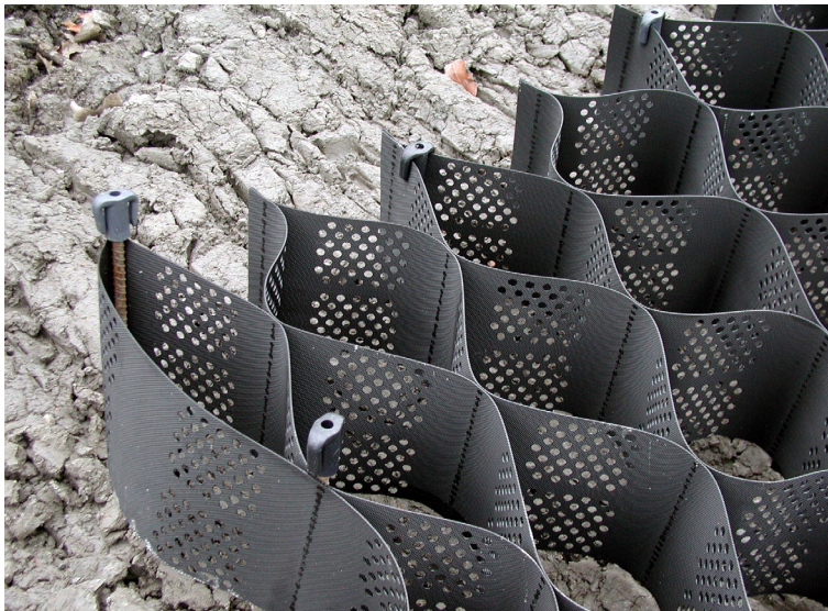
Figure 5. Holes in the cell walls of the Geoweb material allow fibrous roots of native plants to spread from cell to cell and further stabilize shoreline soils.
