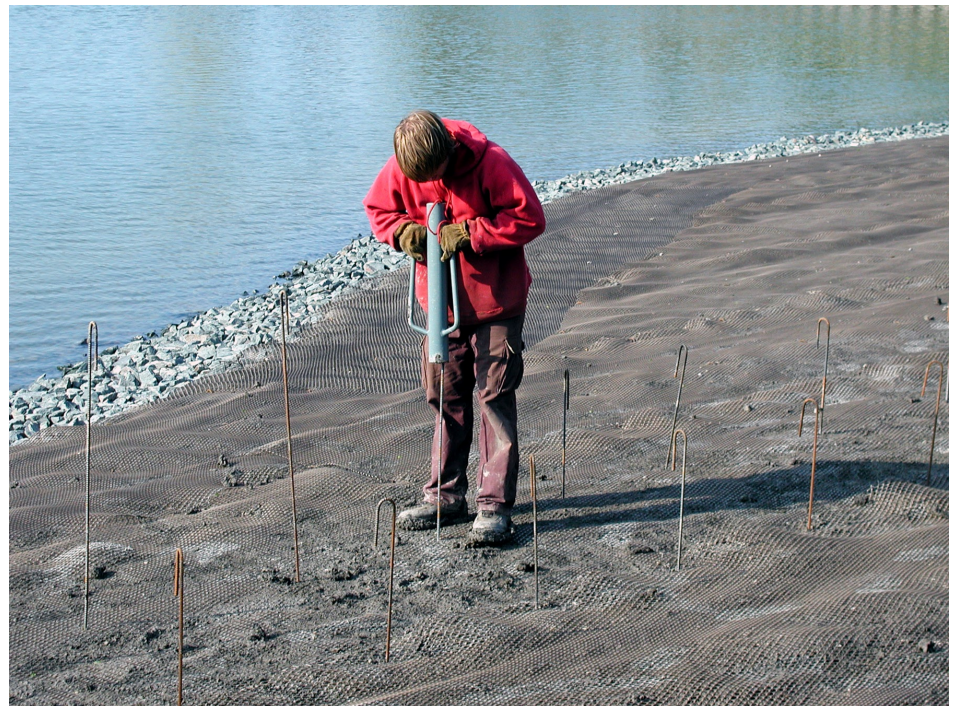
Figure 6. Benthic mesh installed on the lakebed prevents disruption of young plants by carp, and allows foot traffic atop soft lakebeds for invasive species removal in new planting beds (note that the lake level is drawn down in this photograph).
