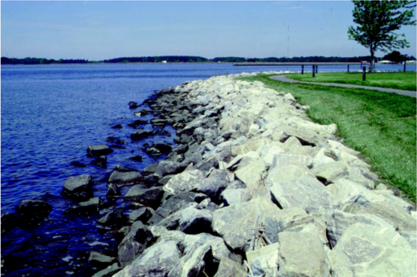
Figure 16-51 Rock riprap revetment
