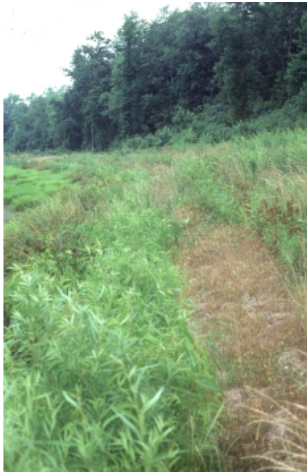
Figure 16-9c An established 2-year-old live fascine system (Robbin B. Sotir & Associates photo)
