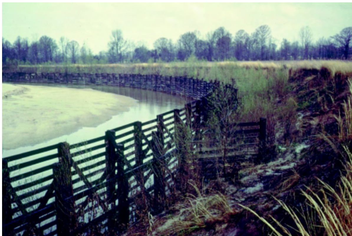
Figure 16-28 Slotted board fence system
