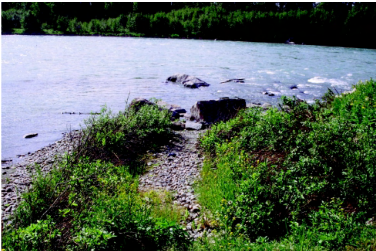
Figure 16-53 Live siltation construction system (Robbin B. Sotir & Associates photo)
