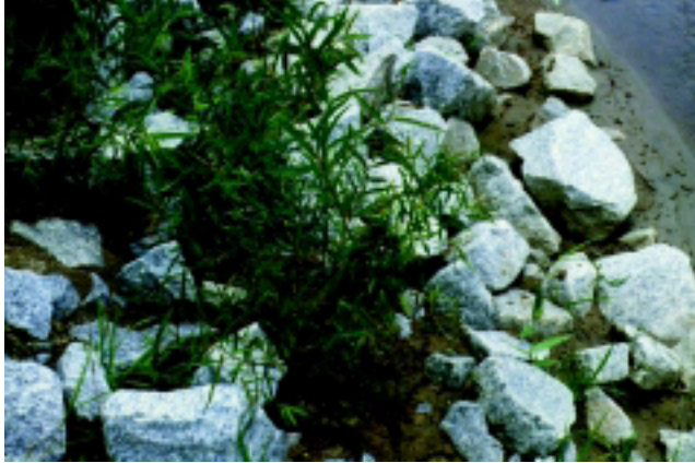
Figure 16-17a Live stake tamped into rock joints (joint planting) (Robbin B. Sotir & Associates photo)
