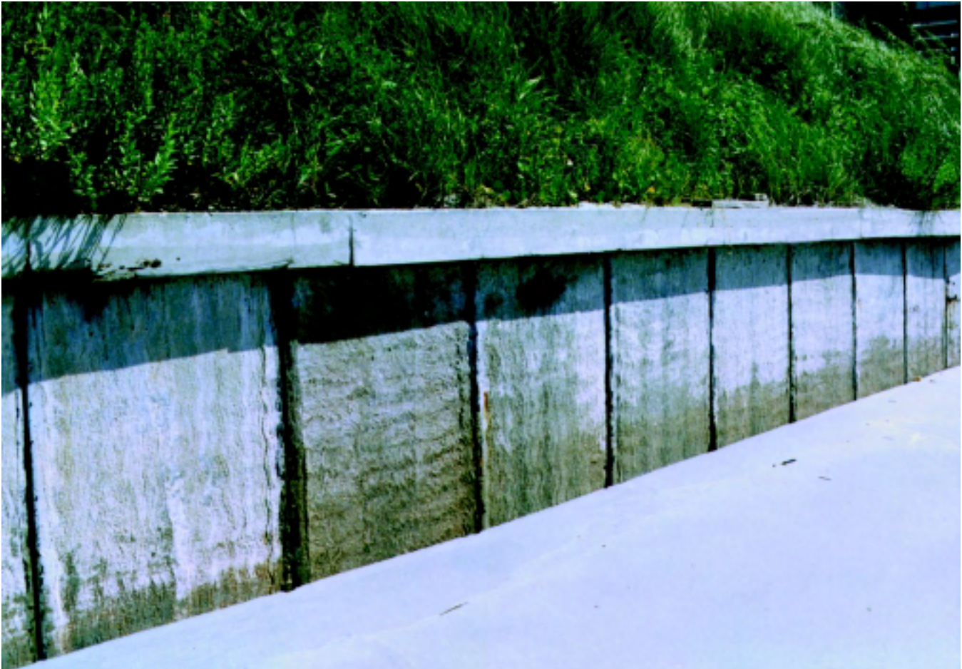
Figure 16-49 Concrete bulkhead system
