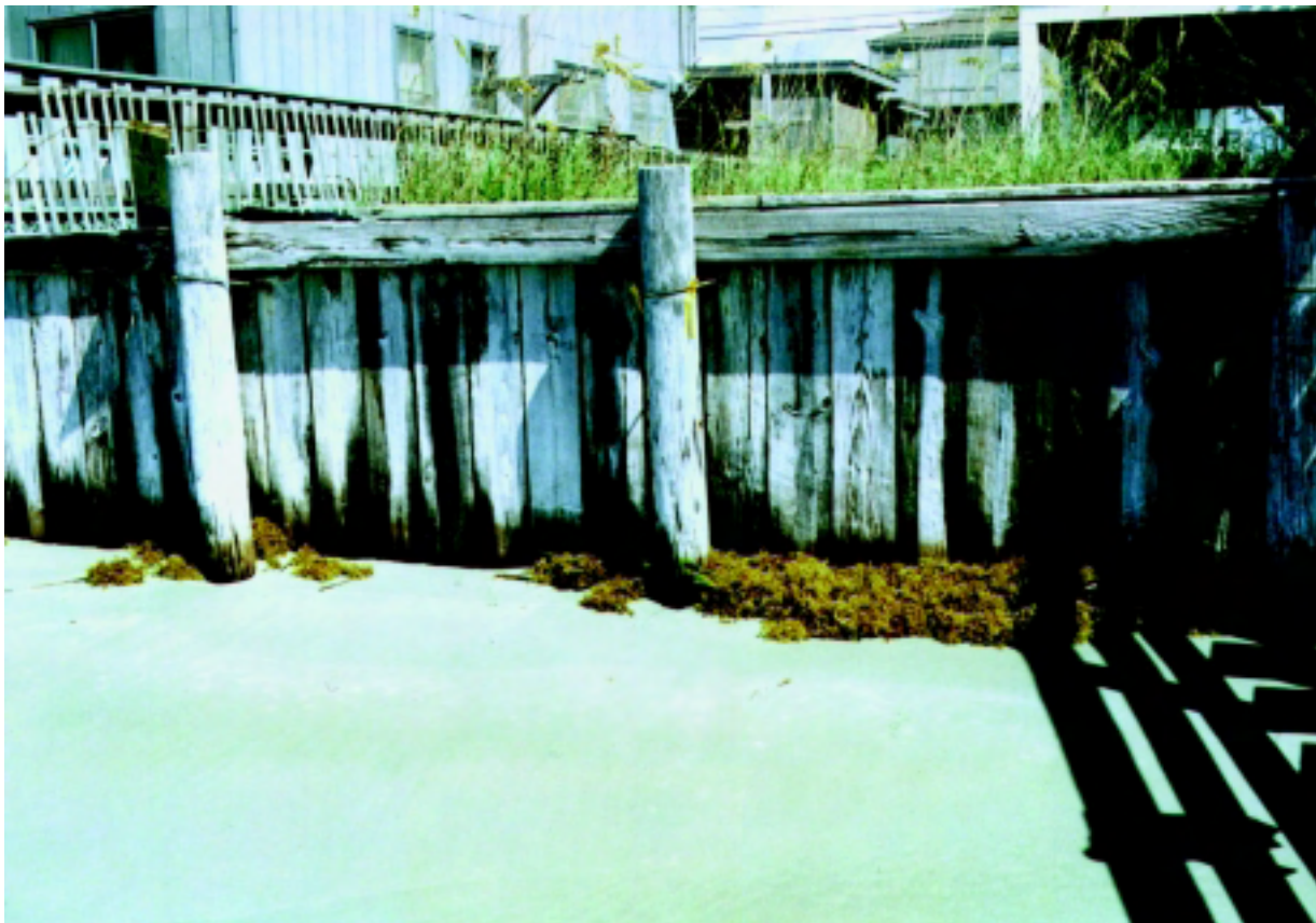
Figure 16-46 Timber bulkhead system
