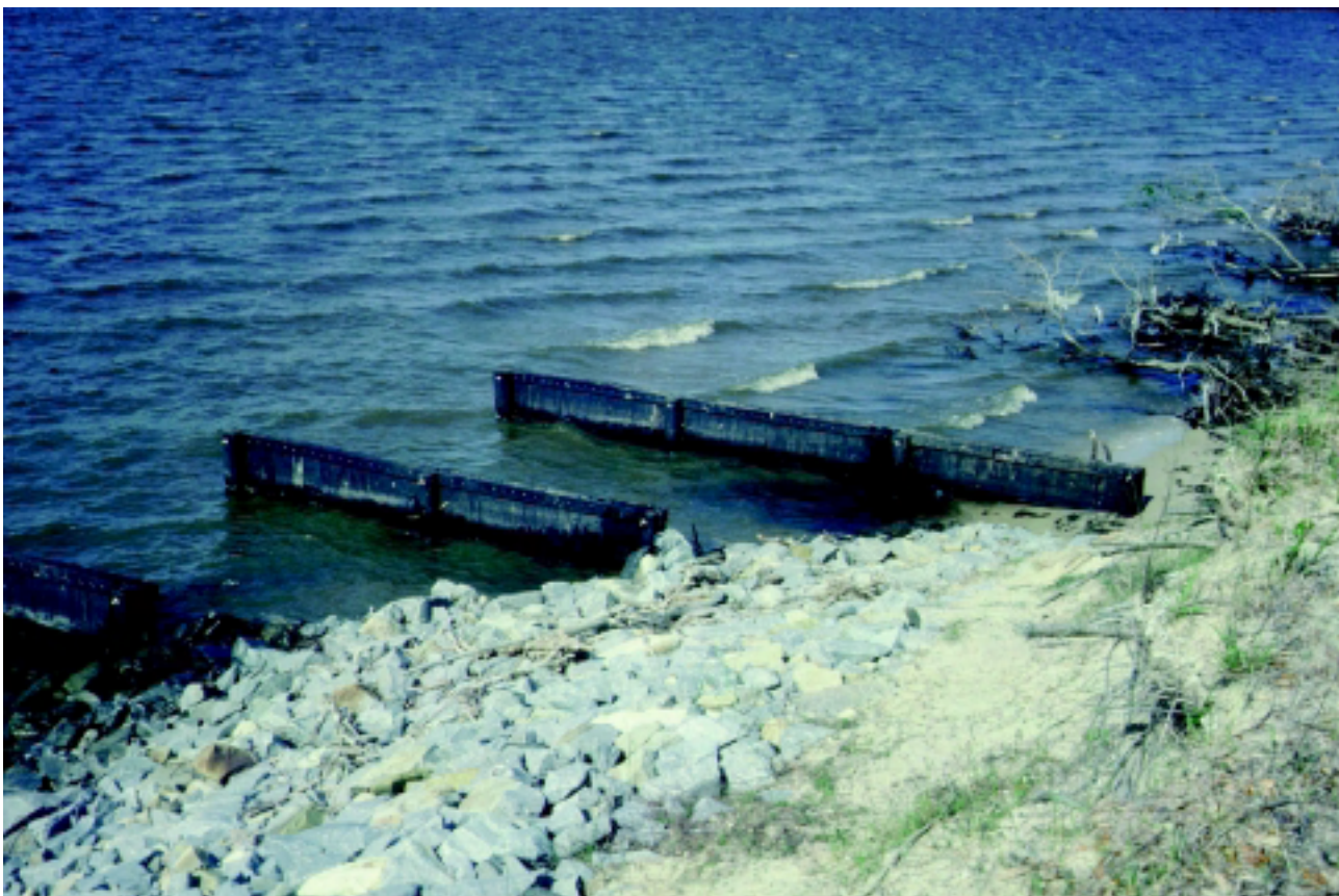
Figure 16-45 Timber groin system
