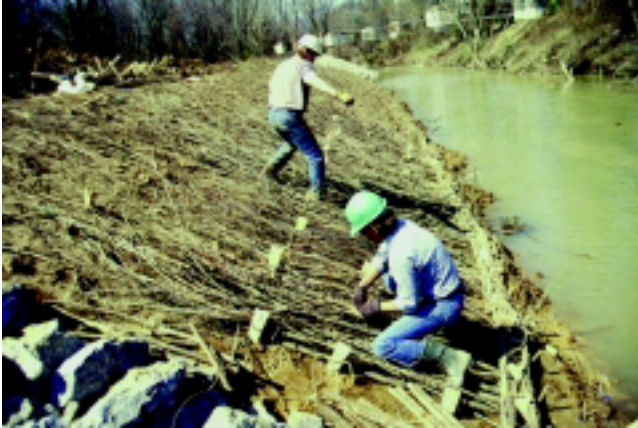
Figure 16-19a Brushmattress during installation (Robbin B. Sotir & Associates photo)
