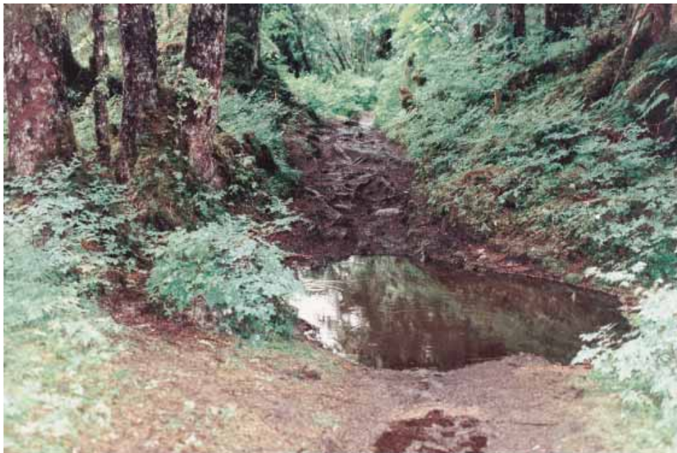
Figure 40—This Alaskan trail is in a rain forest, so it is always wet. Hikers walk on the edges of the trail, trampling plants, ever widening the trail, and exacerbating the problems. The trail is also compacted, muddy, and rutted.
