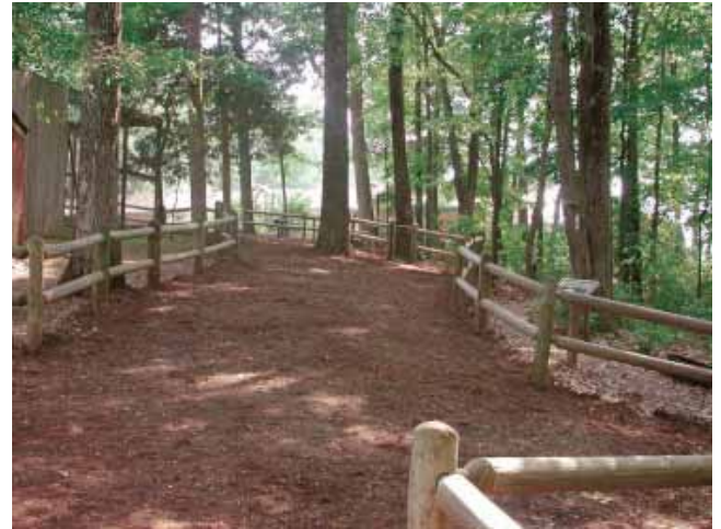
Figure 53—Path is defined by a low fence and is covered in mulch. It is accessible and the mulch protects the soil.
