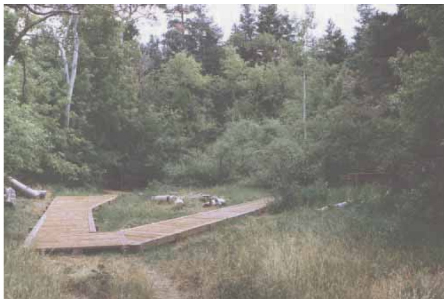
Figure 85—A newly built boardwalk through a trampled meadow.
