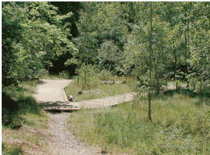
Figure 86—Boardwalk and new vegetation.
