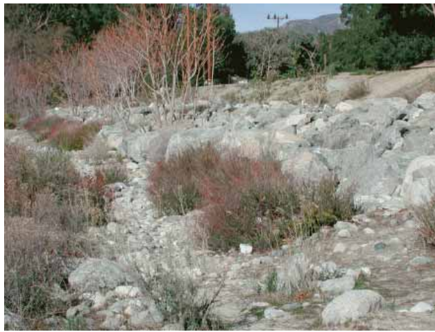
Figure 18—This area was filled to build a parking lot (flat area in upper right) and the bank was stabilized using riprap.
