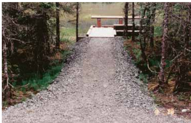
Figure 63—This trail allows water to flow through it, preserving the wetland and providing a dry walking surface.
