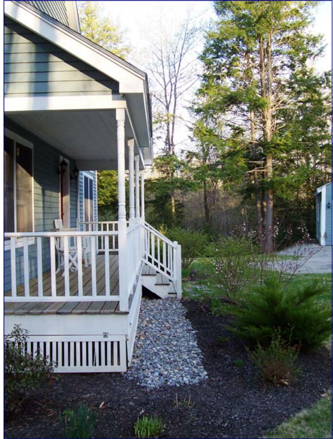
A crushed stone infiltration bed catches and controls roof run-off.
