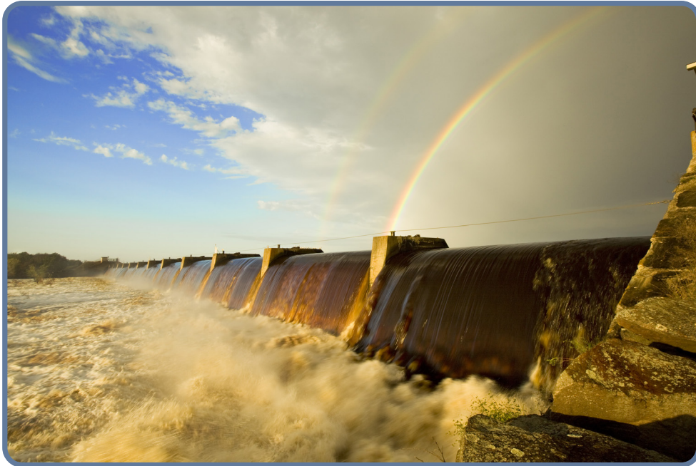
Spillways at Wissota Hydro. Located on the Lower Chippewa River, this facility was completed in 1918 and produces 36.4 MW. Photo Courtesy of Xcel Energy.
