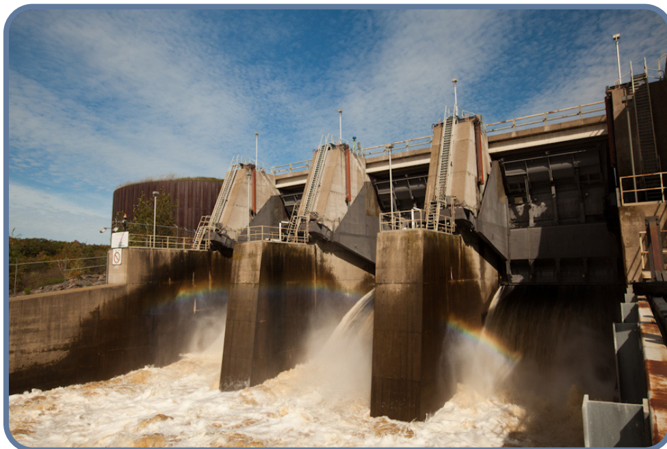
Jim Falls Hydro auxiliary spillway adjacent to the power house. Located on the Lower Chippewa River, this facility was originally constructed in 1923. In 1984, a $92 million redevelopment project made it the largest hydro facility in the Midwest in terms of generating capacity (57.5 MW). Photo courtesy of Xcel Energy.
