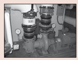
This pump circulates hot water from the boiler room to various parts of the school building.
