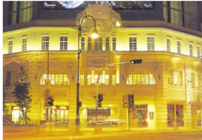
Exterior lighting for night time use should provide adequate visibility
