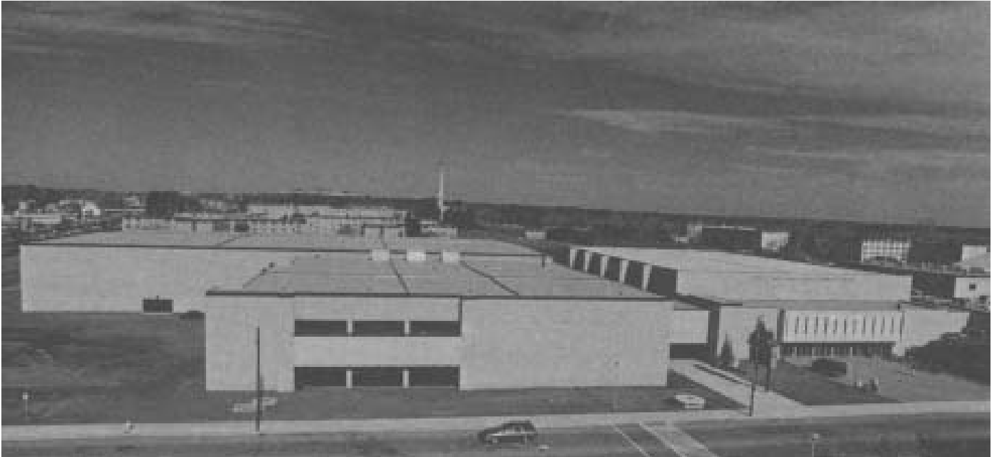
Health Enhancement Center and Quandt Gym at west end of the physical education facility.
