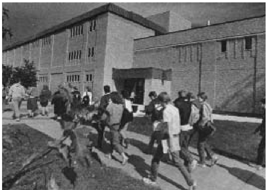
Paper Science wing on the southwest corner of the Science Building.
