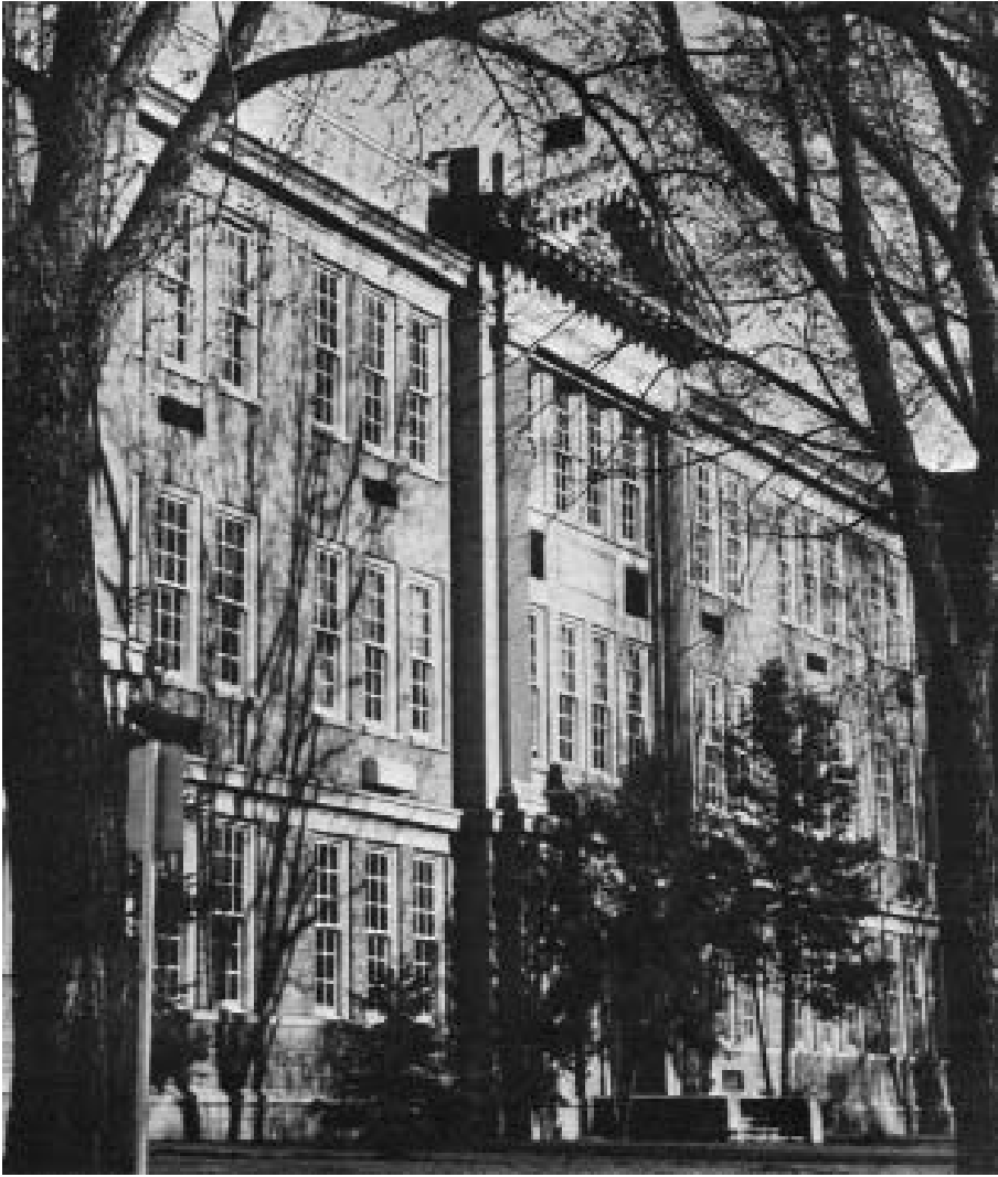
Training School built in 1926; became the Communications Arts Center in 1974.
