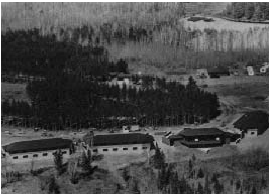
Treehaven field station near Tomahawk while under construction.
