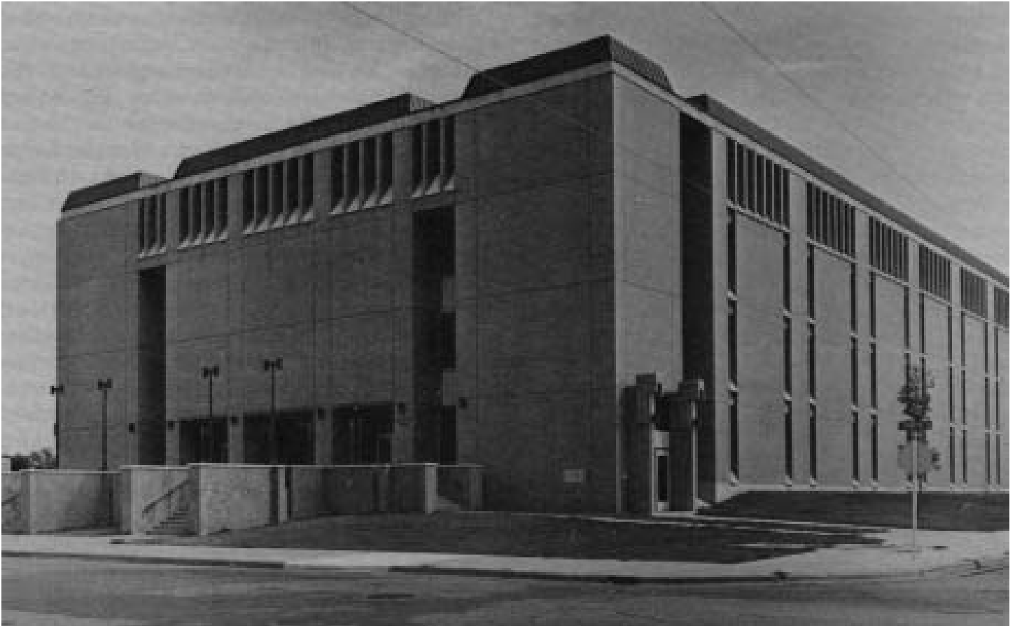
Collins Classroom Center
