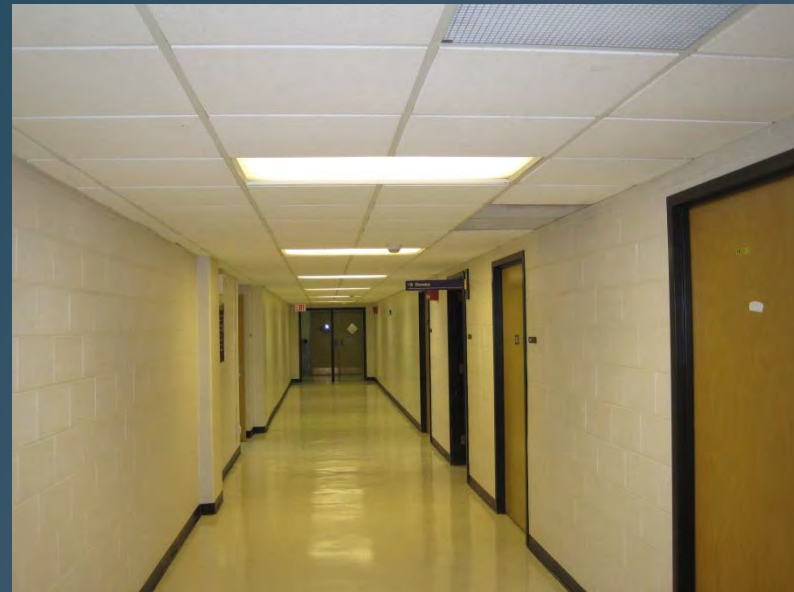
Over Lit Hallway at SSC – Bring Lighting to Correct Lumen Levels
