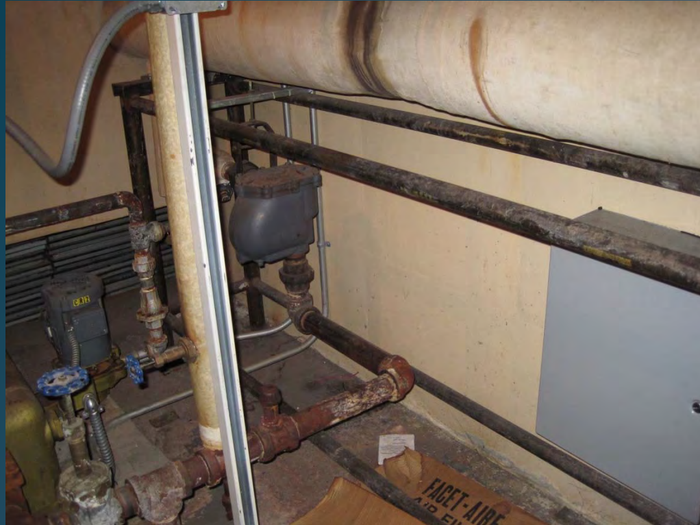
Typical Steam Trap at SSC
