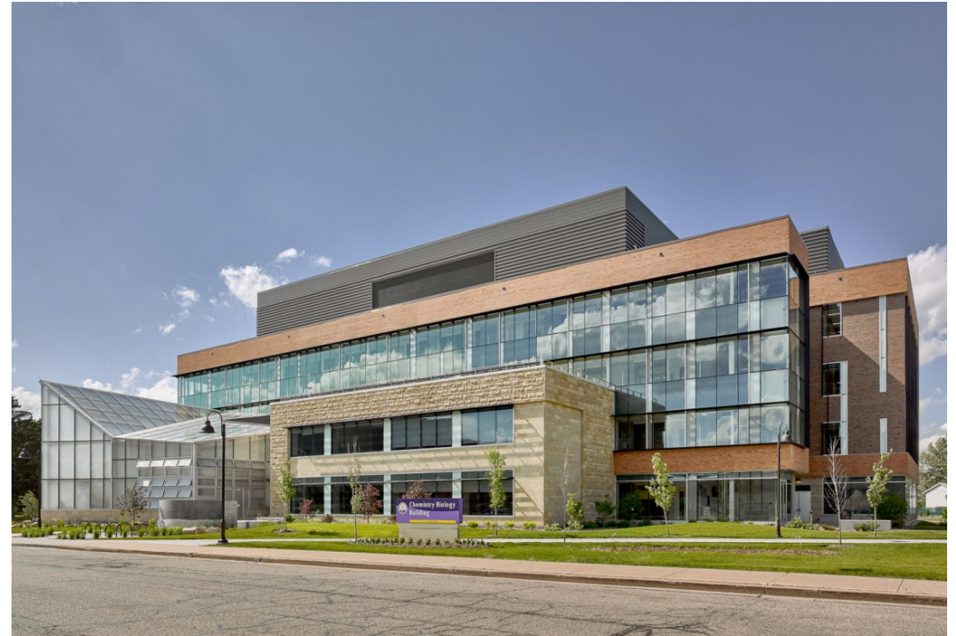
Major Project Example: Construction of the Chemistry Biology Building 2018
