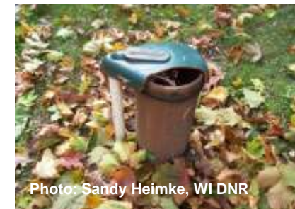
Cracked or poorly sealed well caps can provide insects and other organisms a pathway into your well.
