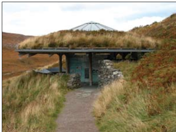
This trailhead structure in Knochan Crag National Nature Reserve, Scotland, harmonizes with the stone and heather of this mountain environment.
