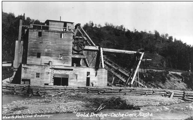
Bucketline gold dredge in the Cache Creek drainage at the base of the Peter Hills, 1931. Locally abundant coal was used for power.
