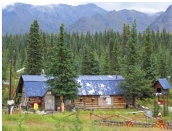
Homesteads in Alaska are creatively constructed of locally available materials. This cabin showcases rough log construction, a metal roof, and a traditional cache. August, 2007
