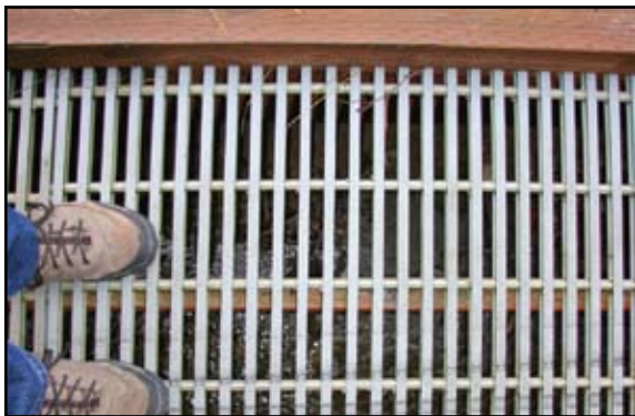
Boardwalks with grate surfaces allow water and sunlight to pass through. Islands & Ocean Visitor Center, Homer
