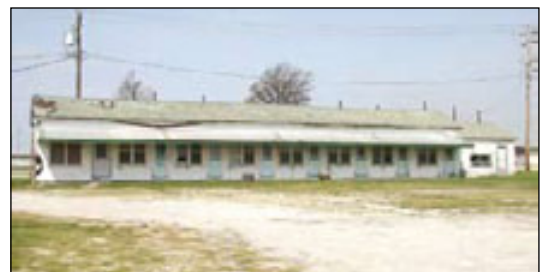
The Belevidere Motel and Cafe in Litchfield is a complex of well preserved buildings along Route 66. April, 2007
