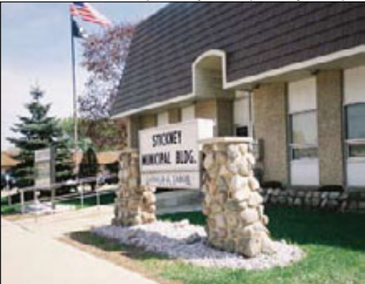
The Village of Stickney Municipal Building.
