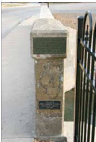
A panel at the 1926 Route 4 bridge in Pontiac could interpret the evolution of road construction and the first hard road across Illinois. March, 2007
