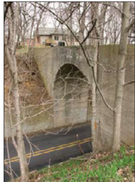
Gillett Memorial Arch Bridge, Elkhart. March, 2007
