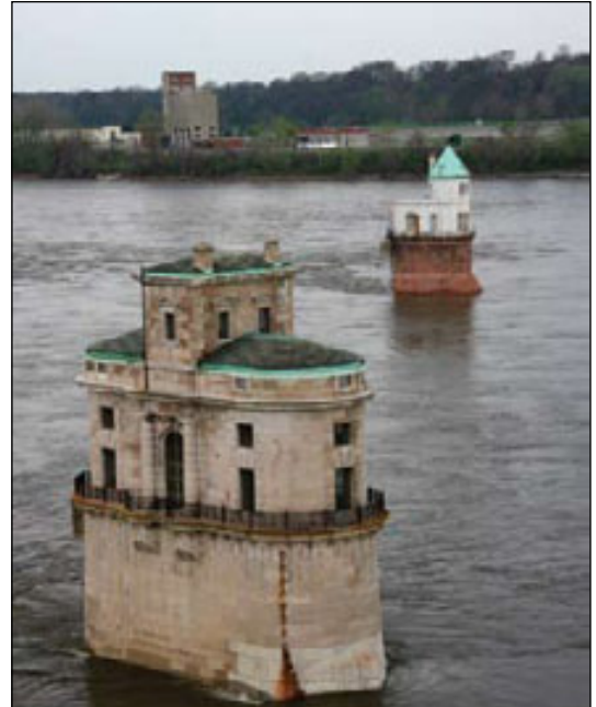
Historic water intake towers from the Chain of Rocks Bridge, Madison. April, 2007
