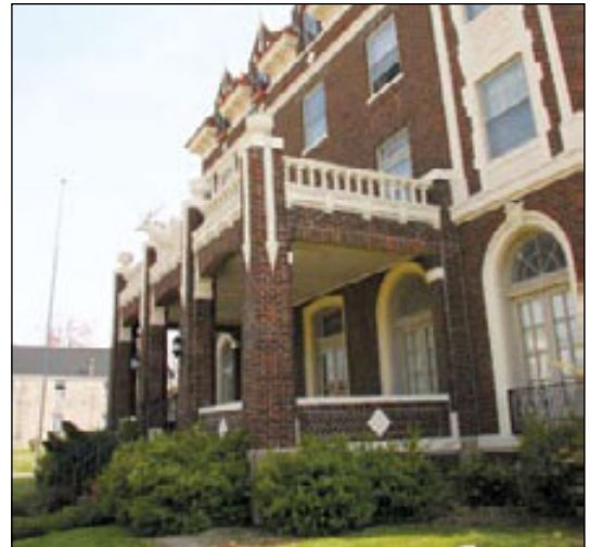
Elks Building, Litchfield. April, 2007
