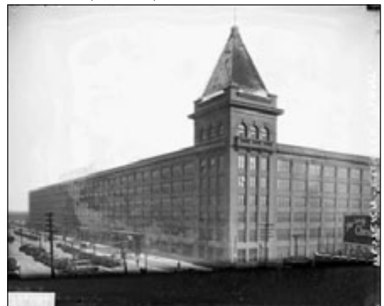
Historic photo of the Western Electric Hawthorne Works, Cicero
