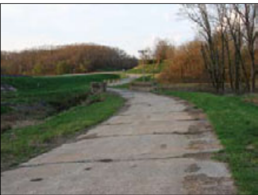
Deerfield Drive original pavement and bridge, south of Carlinville. March, 2007
