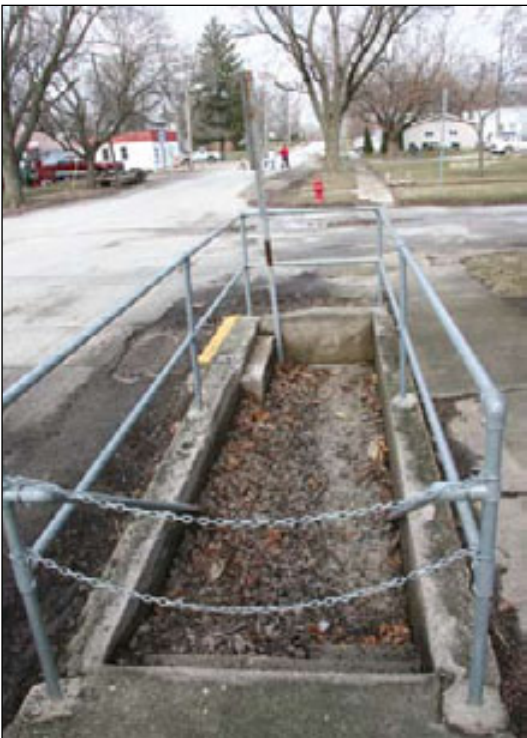
Odell “Subway” Tunnel. March, 2007
