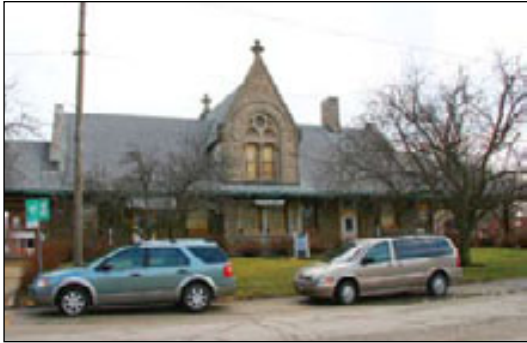
The Dwight Depot offers a commanding view of downtown historic buildings. An interpretive panel here could feature their stories. March, 2007
