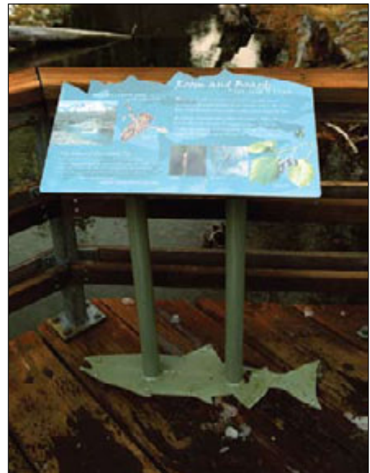
High-pressure laminate is a relatively inexpensive panel material that holds up well to vandalism and the elements. It can be produced in a variety of thicknesses and cut into any shape.
