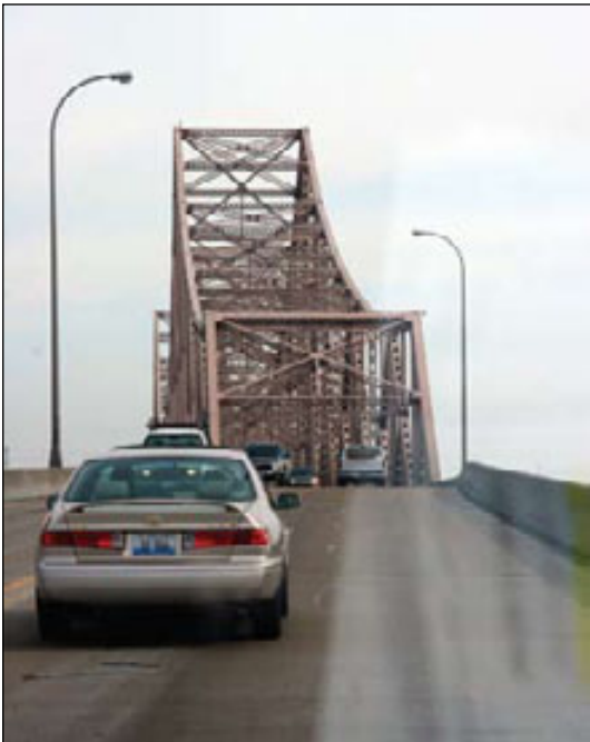
Martin Luther King, Jr. Memorial Bridge, East St. Louis. February, 2008
