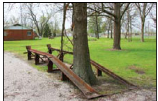
A tree now grows through the Soulsby’s Service Station drive up ramp, Mt. Olive. April, 2007
