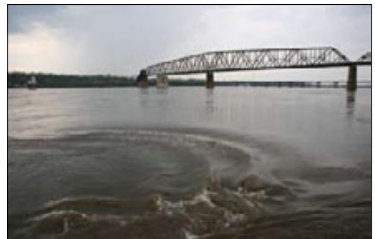
Swirling water rushes over the "chain of rocks." Chain of Rocks Bridge, Madison. April, 2007
