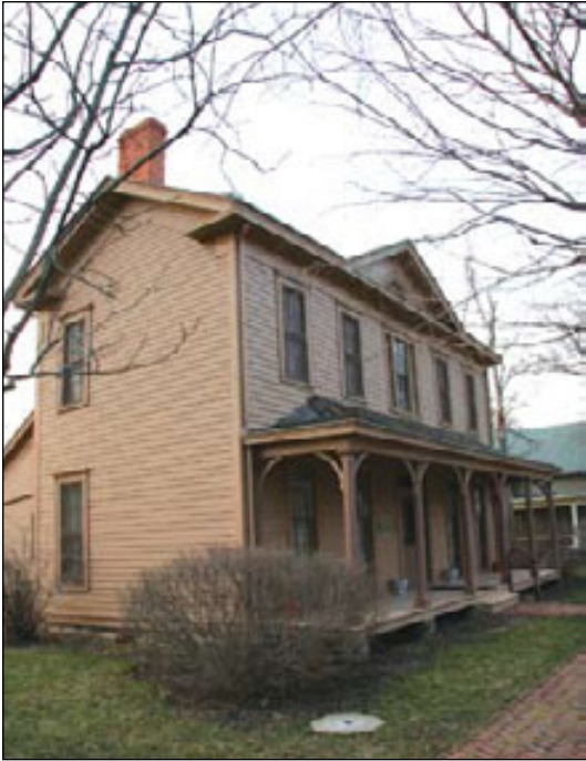
The Matthew Scott home in Chenoa is a beautifully restored historic building. But, without an appointment, visitors can't view the finished interior. March, 2007
