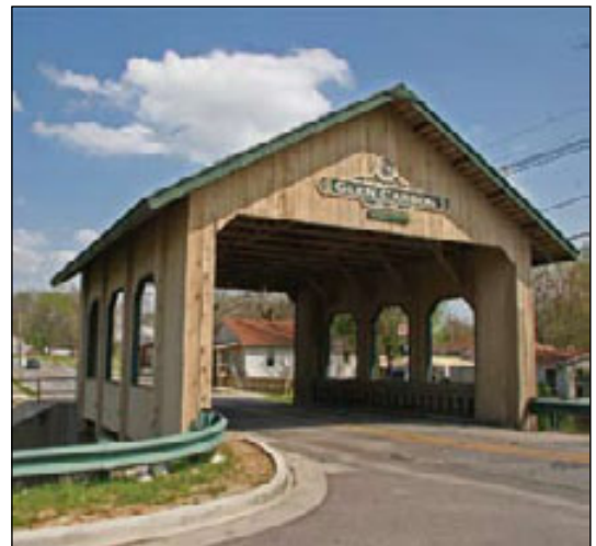
Glen Carbon Covered Bridge. April, 2007
