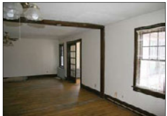
Nominated to the National Register of Historic Places in 2007, Sprague's is probably the largest station/restaurant with living quarters on Route 66. Normal. August, 2007
