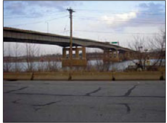
Poplar Street Bridge, East St. Louis.
