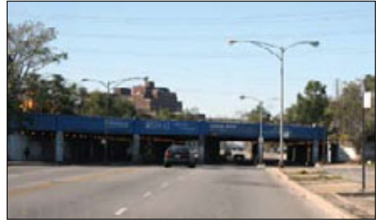
1910 Railroad Viaduct, Chicago. November, 2007
