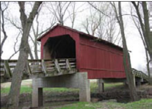
Sugar Creek Covered Bridge, Glenarm. March, 2007
