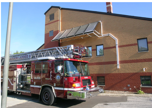
Photo CP4: Solar hot water heaters were installed at Fire Station 6. (Photo courtesy of the city of Madison)
