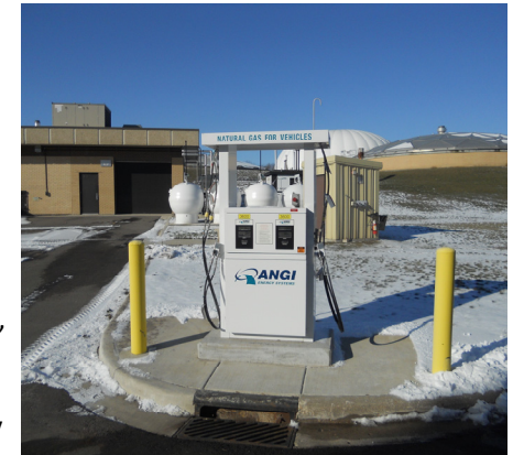
Photo B1: City of Janesville Fast Fill Gas Pump. The Janesville wastewater treatment plant produces biogas (bio-CNG) for use in municipal vehicles. (Photo courtesy of city of Janesville)
