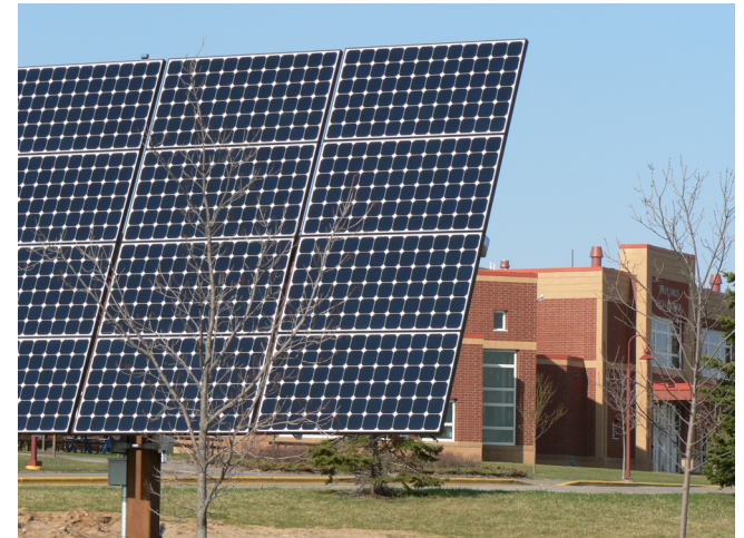
Photo CP3: In 2007, a 3.7 kW photovoltaic dual-axis tracker system was installed at River Falls High School. A kiosk and website provide real-time energy production data. The system provides an estimated 5,236 kWh of energy per year. (Photo courtesy of River Falls Municipal Utilities)
