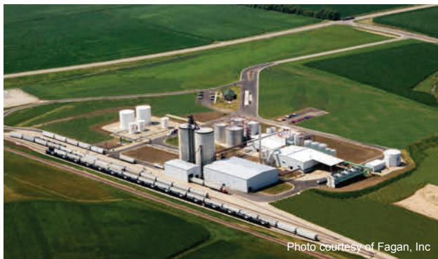
Photo 3 Ethanol facility in Friesland, Wisconsin
